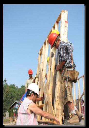
Frame walls are installed, and bales will infill the frames. Post and beam is used on the porch overhangs.
