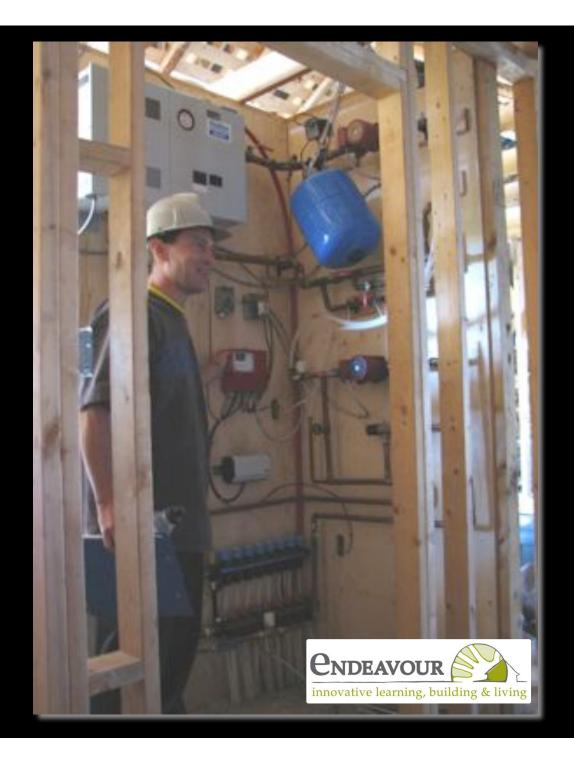
The mechanical room houses the radiant floor heating system, including an electric on -demand boiler, controls, pumps and headers. The controls read outside temperature and activate the system based on temperature changes.
