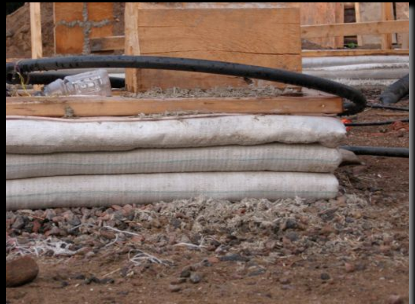
Earthbag foundation with natural stone post footings.
