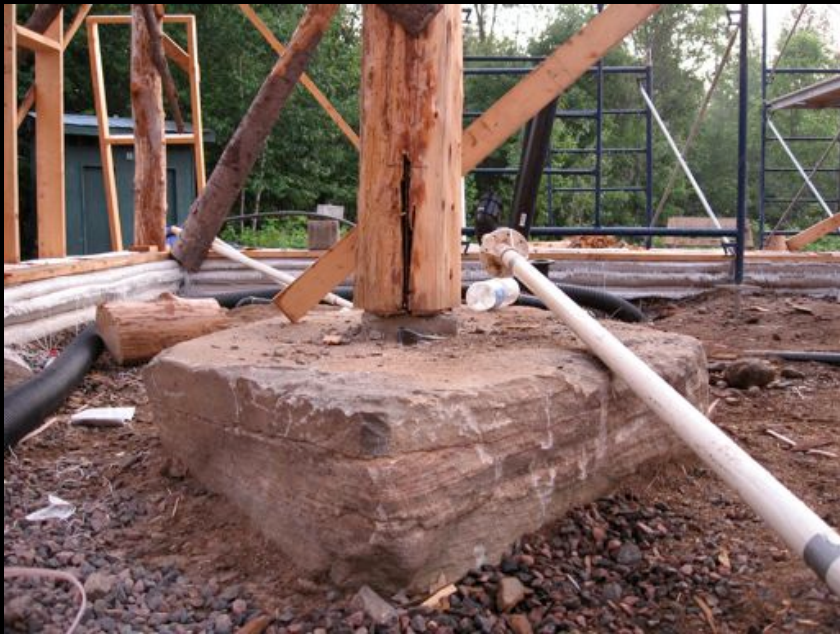
Earthbag foundation with natural stone post footings.
