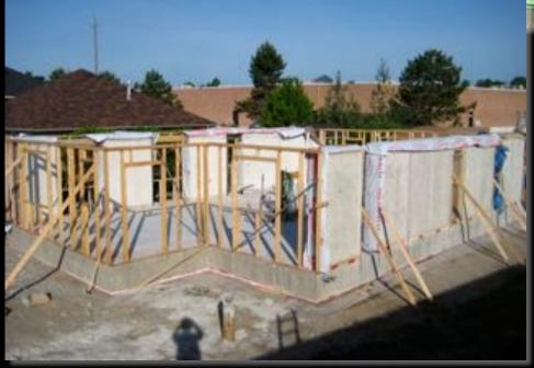
Within a matter of hours, the prefabricated straw bale walls are craned in place and ready for the roof. The walls will bear the weight of the roof.
