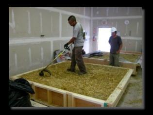
Prefabricated straw bale wall panels are built in a nearby shop and will be ready to install when the foundation is set.
