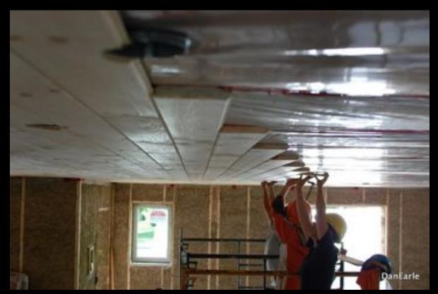
A local pine ceiling is installed, and interior walls are framed. Some are sheathed in magnesium oxide board, others with clay plaster.
