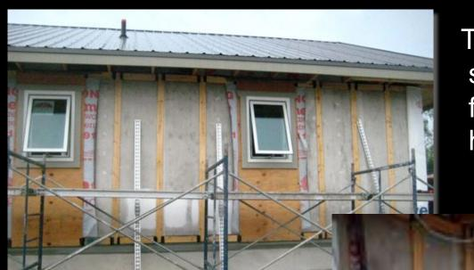
The prefab bale walls are strapped on the exterior for the placement of horizontal siding.
