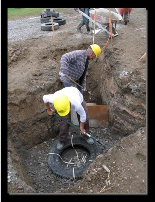
Rammed earth tire piers support the roof posts for the outdoor stage.
