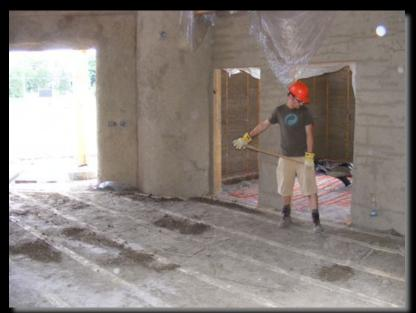
A rammed earth floor base covers the main room, with radiant heat tubing encased. Wooden runners support a floating bamboo floor. Moisture damage from the still damp earth required the bamboo to be replaced.
