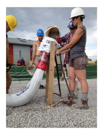
The bag is bunched on the cardboard tube and inserted into the bottomless bucket, and is ready for loading.
