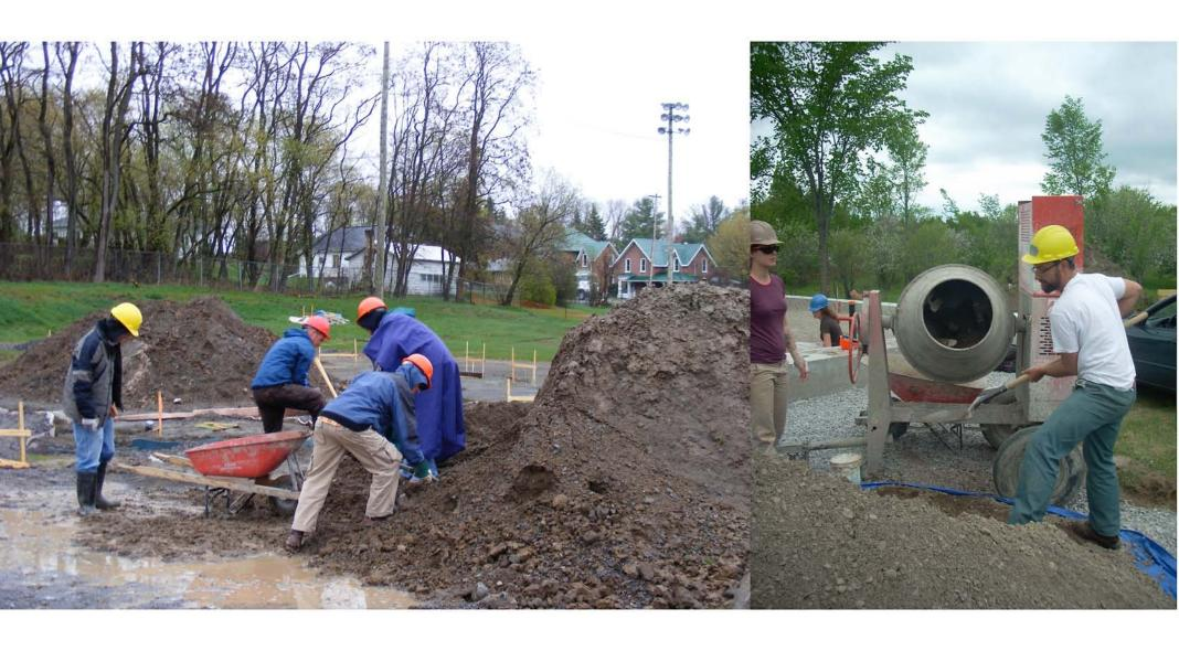
Fill is prepared in barrel-style cement mixer. Mixes should be just damp enough to bind together when tamped. The recipe on the right features crushed stone (40 shovels), hydrated lime (2.5-3 shovels) and metakaolin (2.5-3 shovels) plus a small amount of water.
