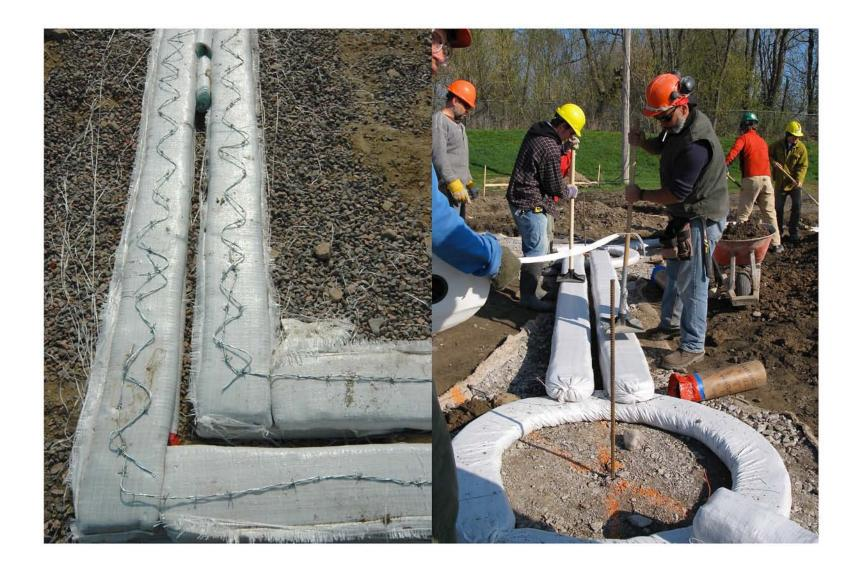
Double wide courses of narrower earthbag can be used to accommodate wide wall systems, and provide space for thermal insulation within the foundation.
