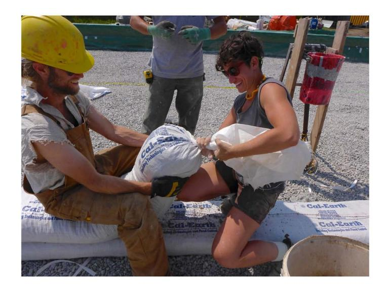
Once the right amount of fill and tamping have been set, the team progresses forward until the end of the bag length or curse. The end of the bag is then twisted off and tucked underneath.
