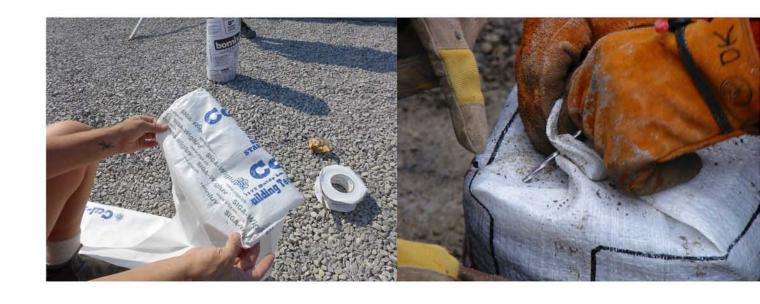
(Left) Wide bag material is sewn to make custom width bags. Ends of bags are folded to create square edges. While not necessary, the work is cleaner and easier to finish this way.
