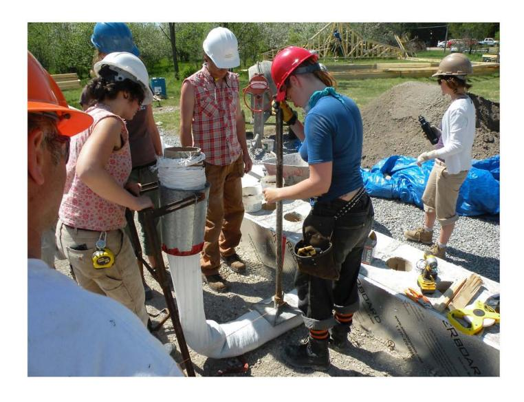
Although it involves some physical labour, we have worked with numerous teams to achieve bag placement rates of 25-30 feet per hour. It compares very favourably with the labour time required to work with concrete at a fraction of the environmental impact and cost.
