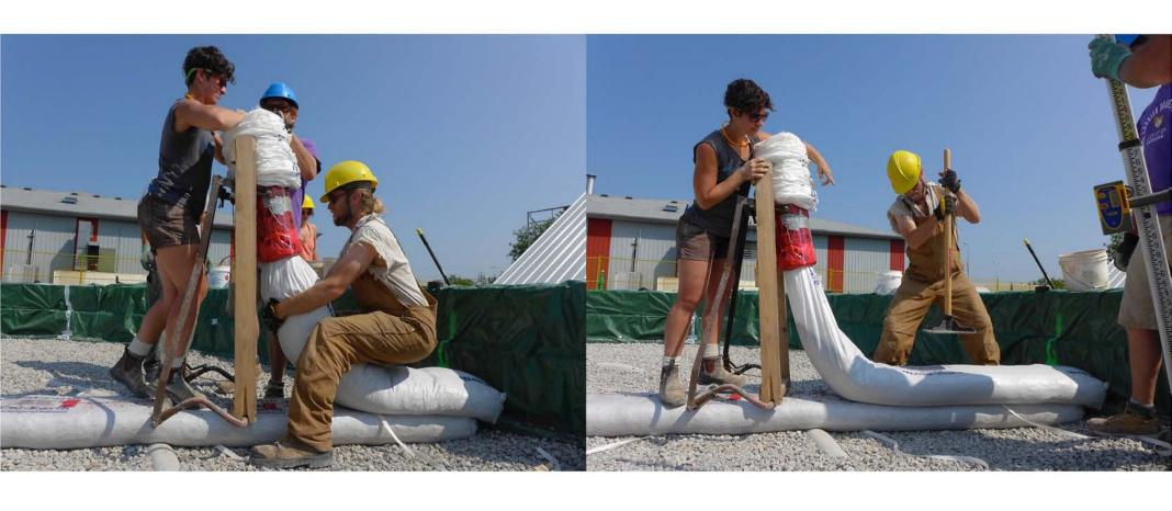
At the start of a course, the desired amount of fill is scooped into the tube via coffee can or bucket. Once filling has proceeded a few feet, the fill is firmly tamped. A height measurement is taken to ensure that each course is the proper thickness.
