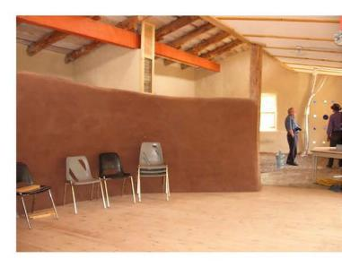
This curved interior earthbag wall is used as both a room divider and also the central heating "radiator". Hydronic tubing is run in the dimples between courses ahead of plastering, and the finished wall provides a steady thermal mass for heating the space.
