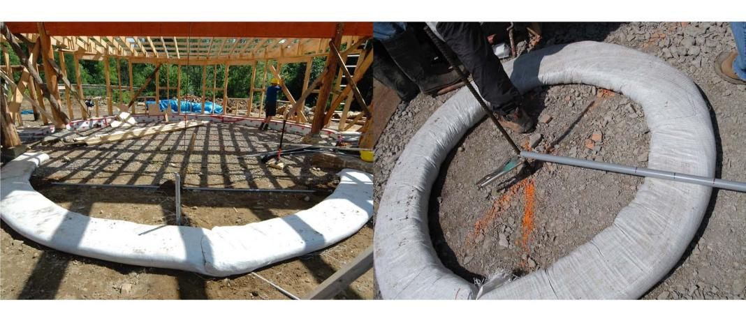
Curved shapes are very easy to create with earthbag. The forming process is much simpler than with any other building system.
