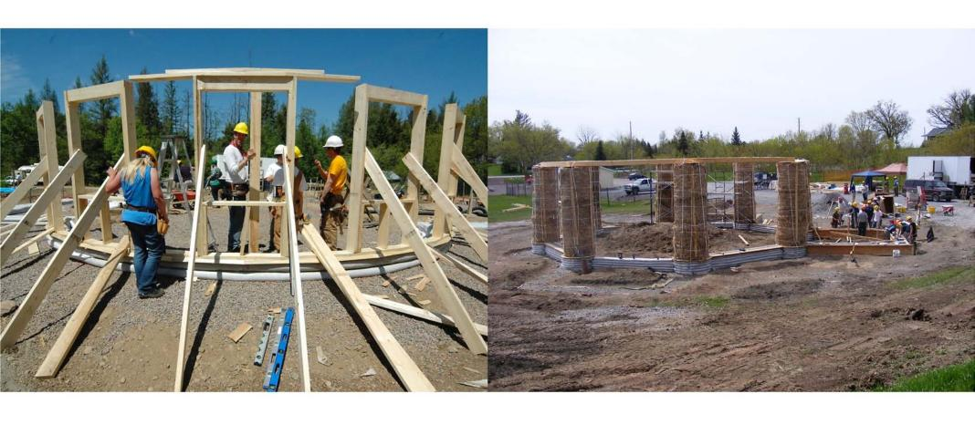
Any type of building can rest on an earthbag foundation. We've used conventional frame walls, straw bales, hempcrete, straw clay and even round straw bale columns.
