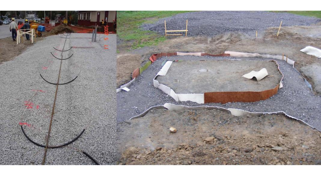
A rubble trench or other stable gravel pad makes an ideal base for an earthbag wall or foundation. The tubes on the left are for compression straps for a load bearing straw bale wall
