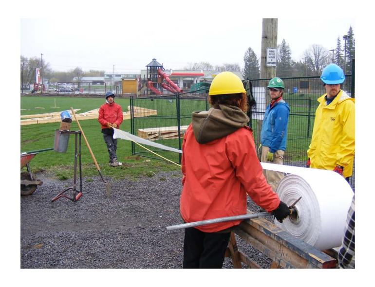
Woven polypropylene bag material can be purchased in continuous rolls, as well as in sewn bag form. Many sizes are available to make different foundation widths.
