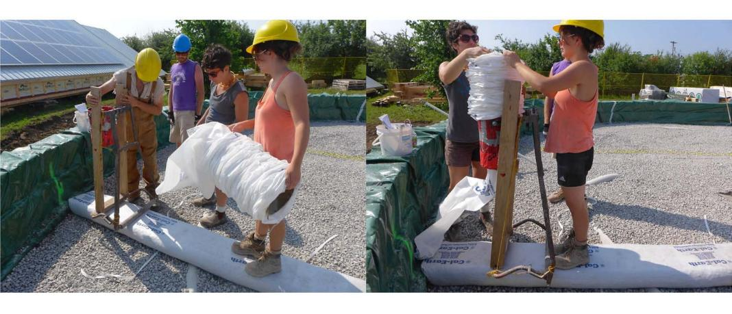
A simple loader is constructed to provide a movable stand that holds a long length of bag. The bottom of the metal bucket is removed, and a cardboard tube fit inside it. The friction fit between the two allows baggers to feed the exact amount of bag required.
