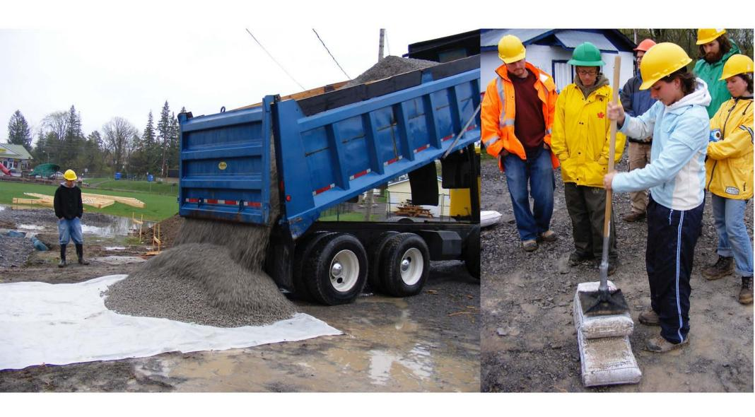
A crushed stone is often used to supplement site soil or to form the basis of a mix. Mixes range from typical concrete mixes to pure gravelly sub soil to those with custom binders. Small test bags can be made to refine recipes.
