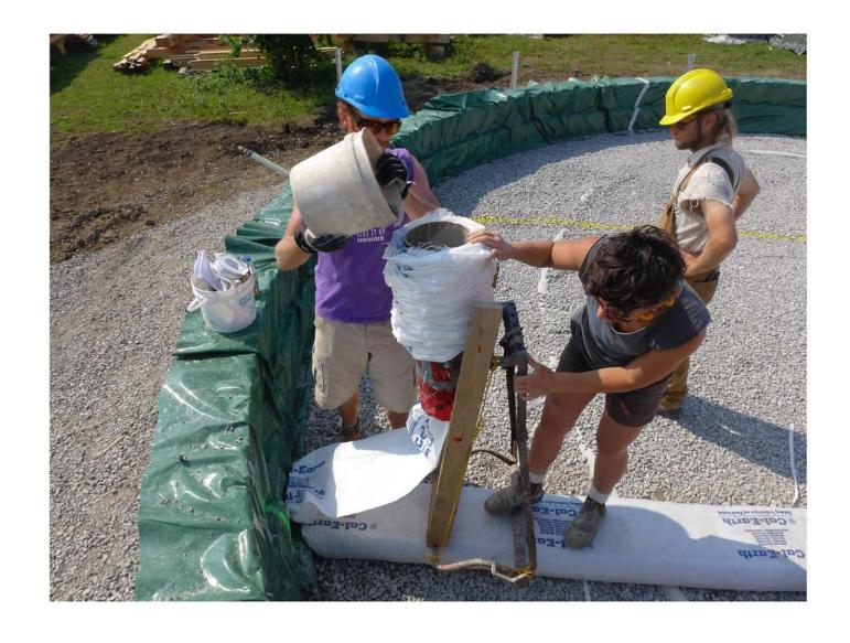
To begin a course of earthbag, the loader is put in place with a desired length of bag. The end of the tube has been squared and properly placed on the foundation line.
