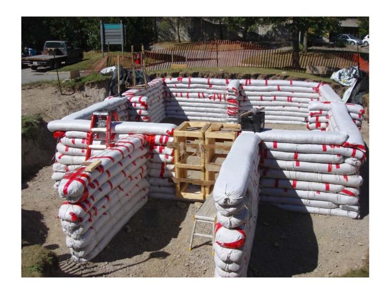
Taller walls, especially those being buried and carrying soil pressure, may require buttressing as seen at the mid-span point of these basement walls.
