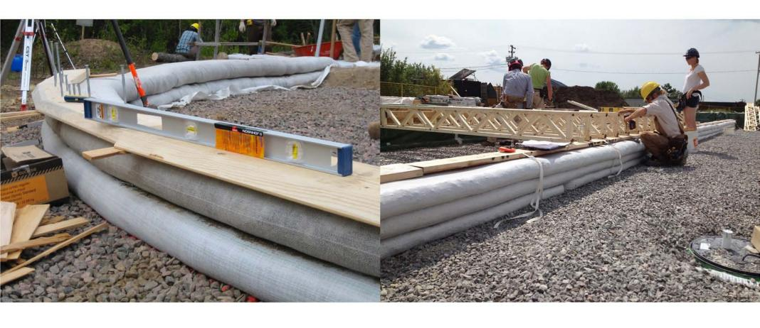
Wooden sill plates are commonly spiked or strapped to earthbag foundation walls to provide attachment for wall systems or floor framing.
