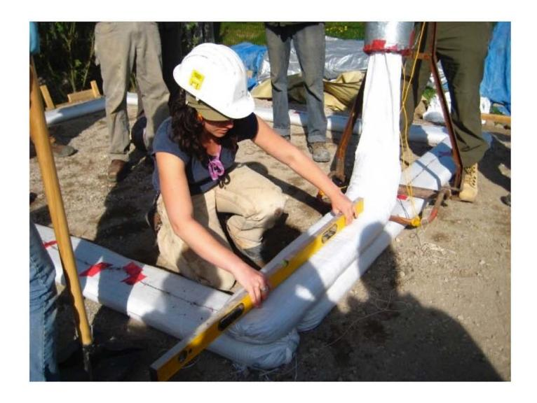
Corners are staggered between courses. The process of checking level is important. Typically, refinements to level are made with each subsequent course until the final course is perfect.
