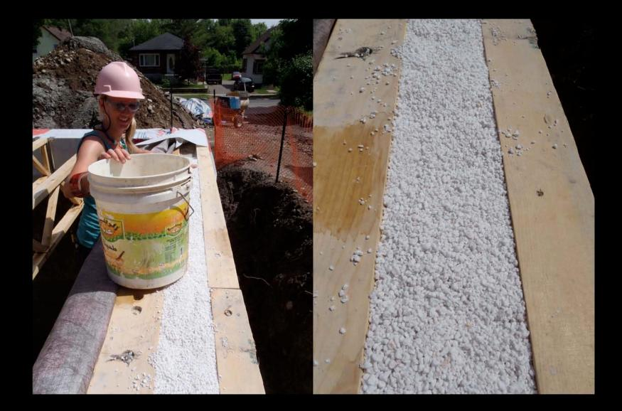
Perlite insulation between sill plates
