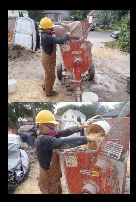
The clay plaster is a stiff mixture that is very high in chopped straw. This allows the entire desired thickness to be installed in one coat, while building up to a very straight and smooth finish.
