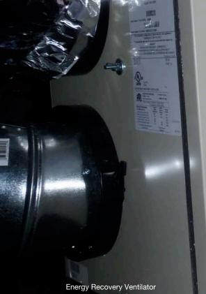
The ERV is a requirement for an air-tight home. It draws fresh air from outside and transfers both heat and humidity to the incoming air from the outgoing air. It keeps the air fresh and balanced in the home. Gold Series
