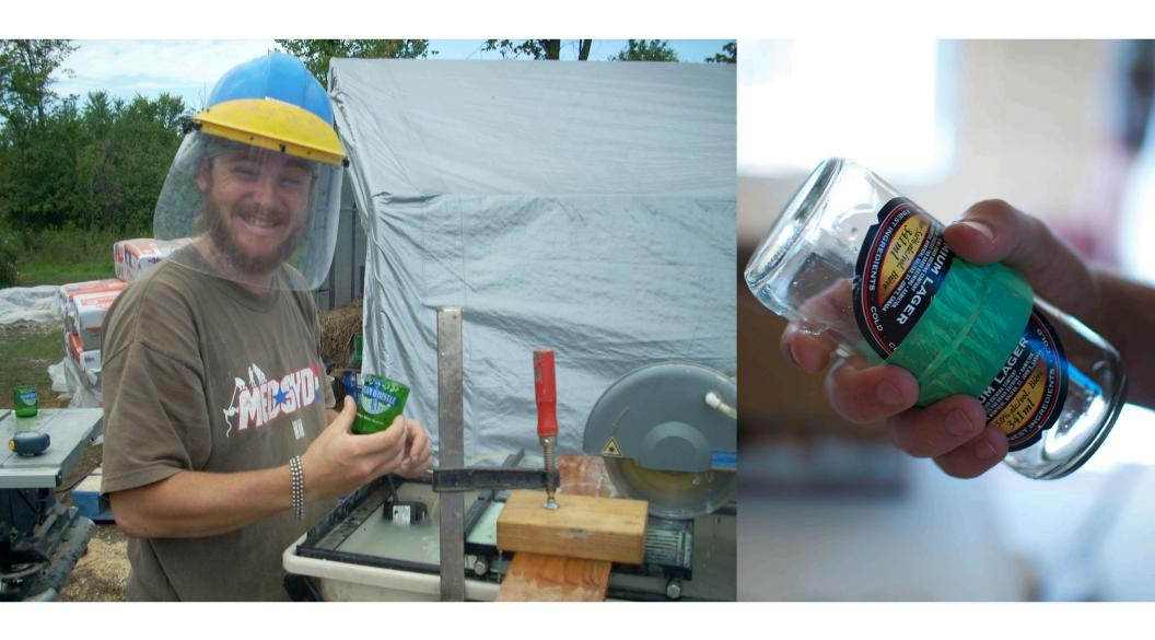
The first step in making a bottle wall is to cut the bottles to the appropriate length. To enable light to pass through the bottle, two bottoms are attached together. Each bottom should be half the desired depth for the intended wall type.
