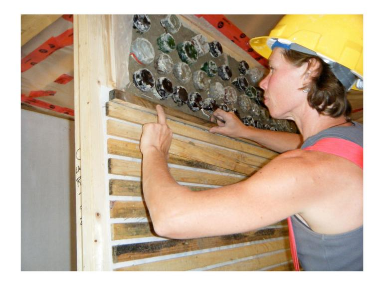
In a straw bale wall (left), the bottles must protrude far enough from the bale (I inch should do) that the finish plaster can be applied around the bottles. "Pointing" around the bottles gives a smooth final finish to the mortar.
