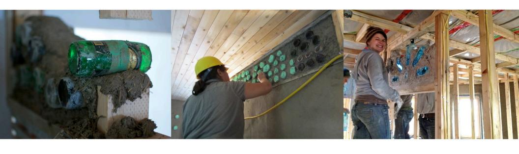
Mortar for a bottle wall can be made from many materials, including cob (straw/clay/sand), hempcrete (lime, chopped hemp) and cementitious mortars.
