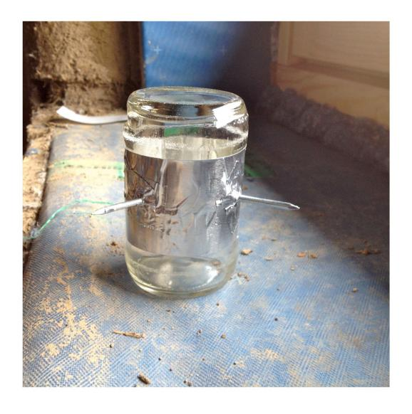
Silver, metallic duct tape works well and is reflective on the inside to help light continue through the bottle. If the bottle is going into a wall material that may not bind well with the glass, nails can be taped to help lock the bottle in place.
