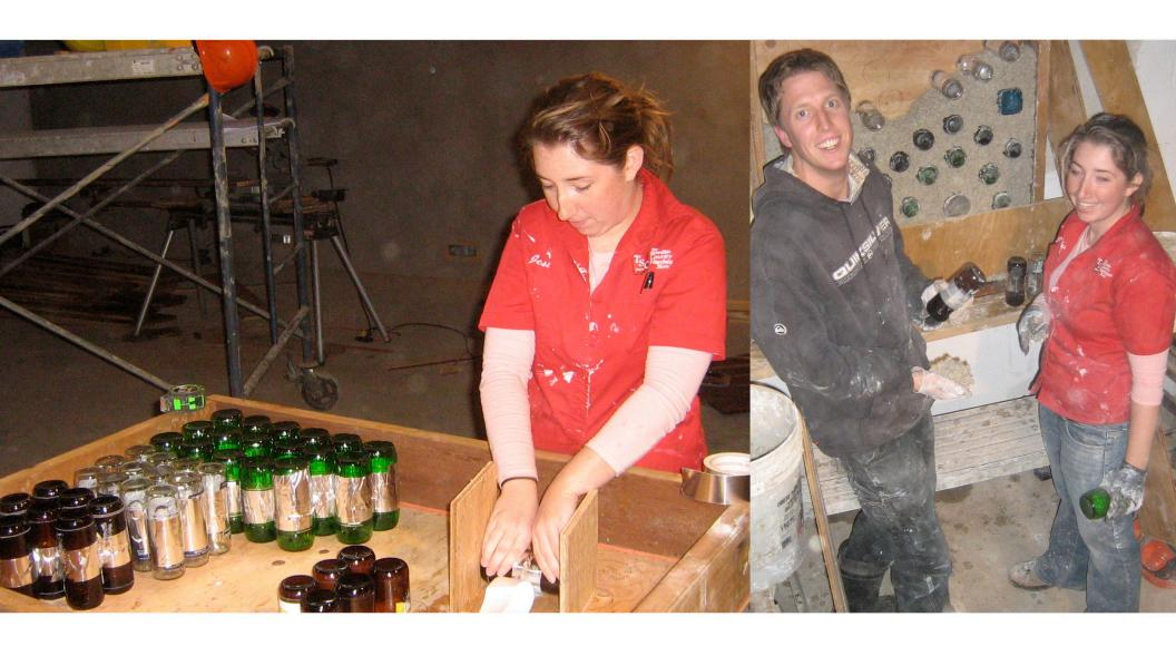
In this case, the bottle wall is being constructed in a form and will be put into place in the wall once it is completed.
