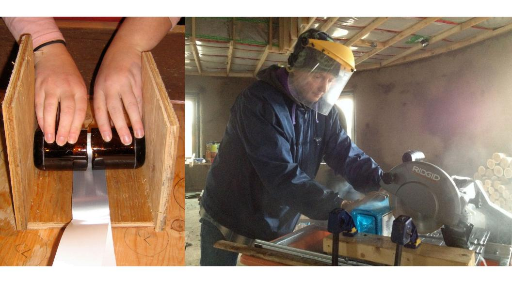
A wet tile saw with a diamond blade is the easiest way to cut the bottles. I hese saws can be rented at most tool outlets. Once cut, the bottles are taped together to make one piece. The bottles should be between 1/2-2 inches wider than the wall they are going into.
