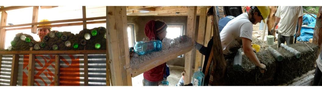
Different wall widths require different layouts and bottle lengths. The frame wall on the left is thin, and bottles are transverse in the wall. Bottles go in line with the frame wall in the centre. On the right, long bottles pass through a wide straw bale wall.
