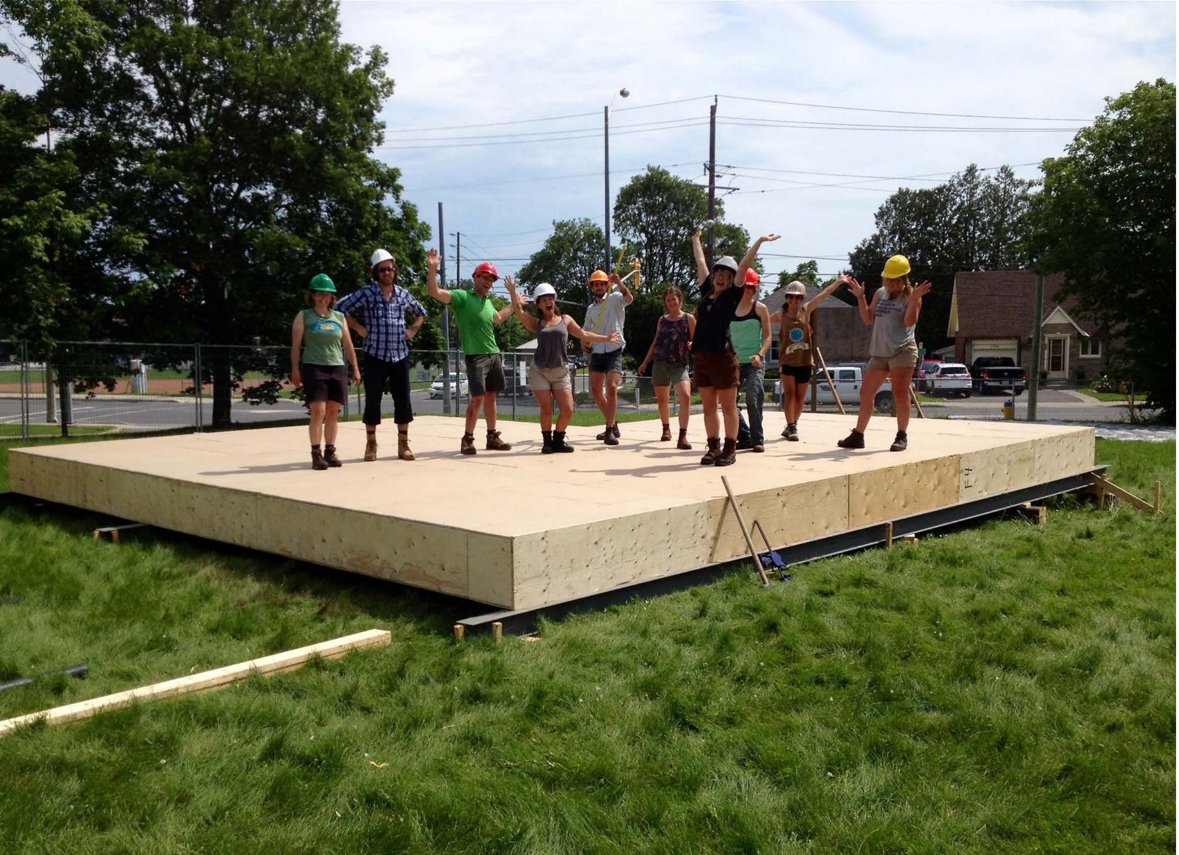
The floor is ready. The five panels come together quite quickly.
