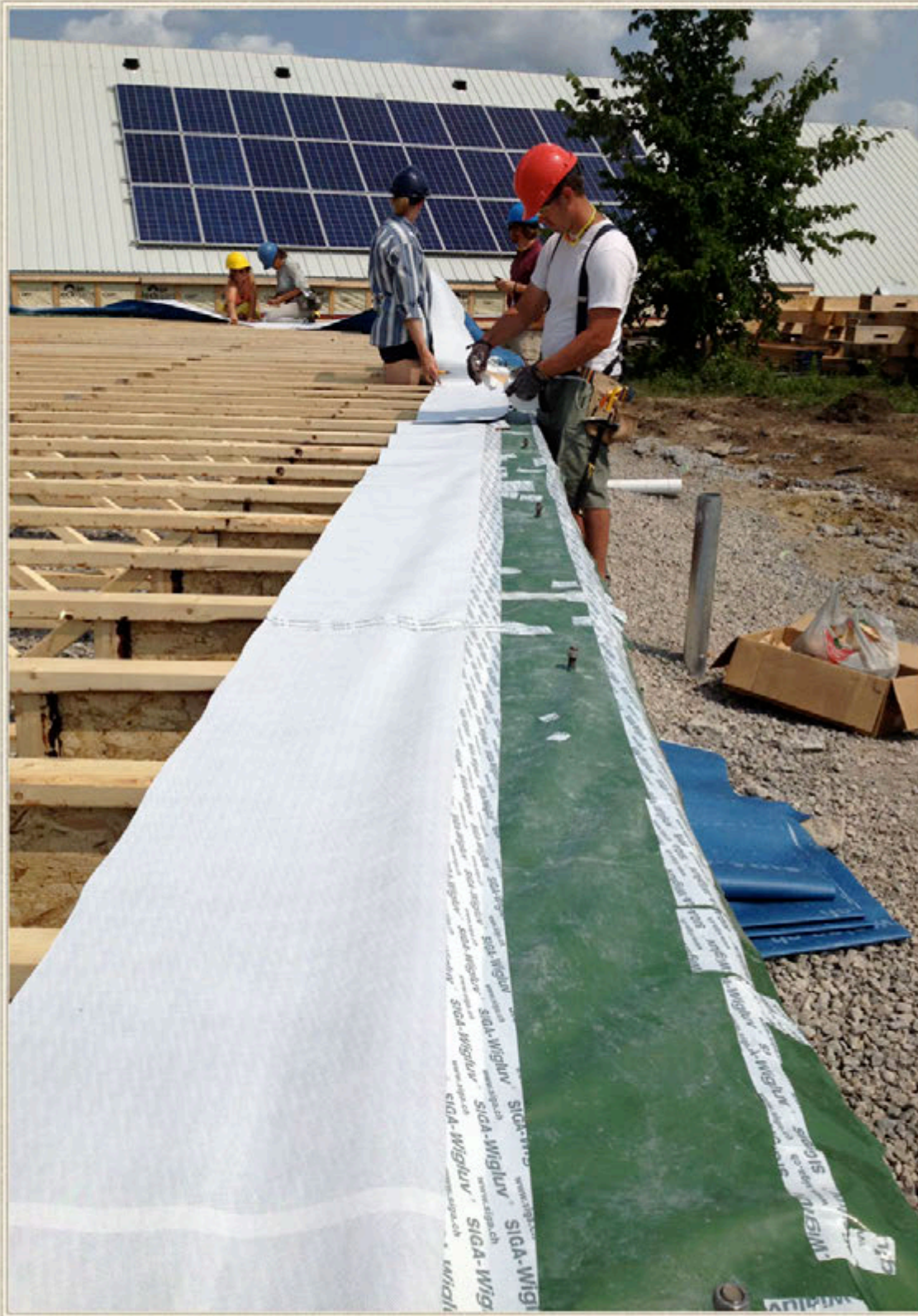
Open web floor joists rest on the Durisol ledge and the earthbag foundation. The vapour barrier is carefully tied in so it joins to the exterior walls.
