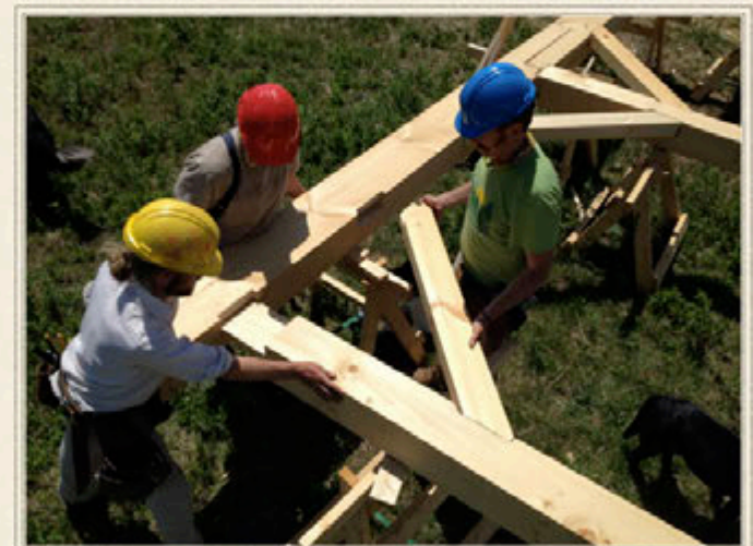
Site work begins with building the four timber frame sections for the corners of the building, using locally harvested and milled white pine timbers.
