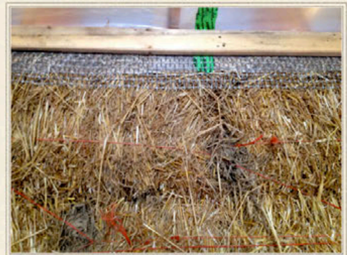
Detailing includes stuffing and lashing joints and taking care of air sealing at all seams using air barriers and mesh.
