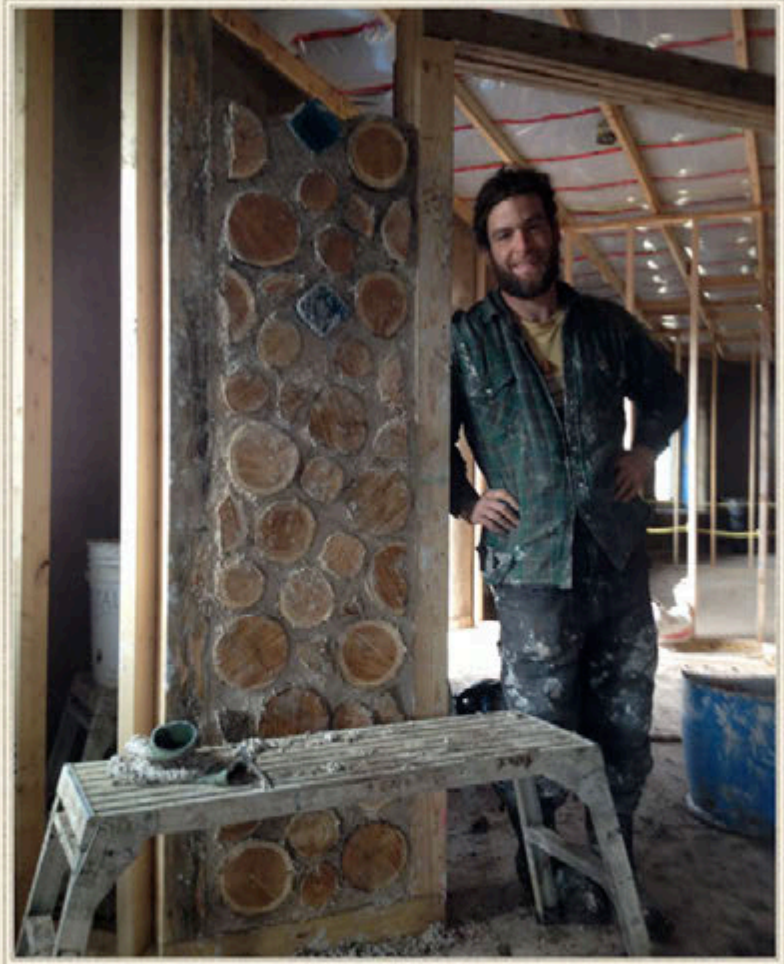
Hempcrete is also used to create a cordwood and bottle entryway to the main meeting room.
