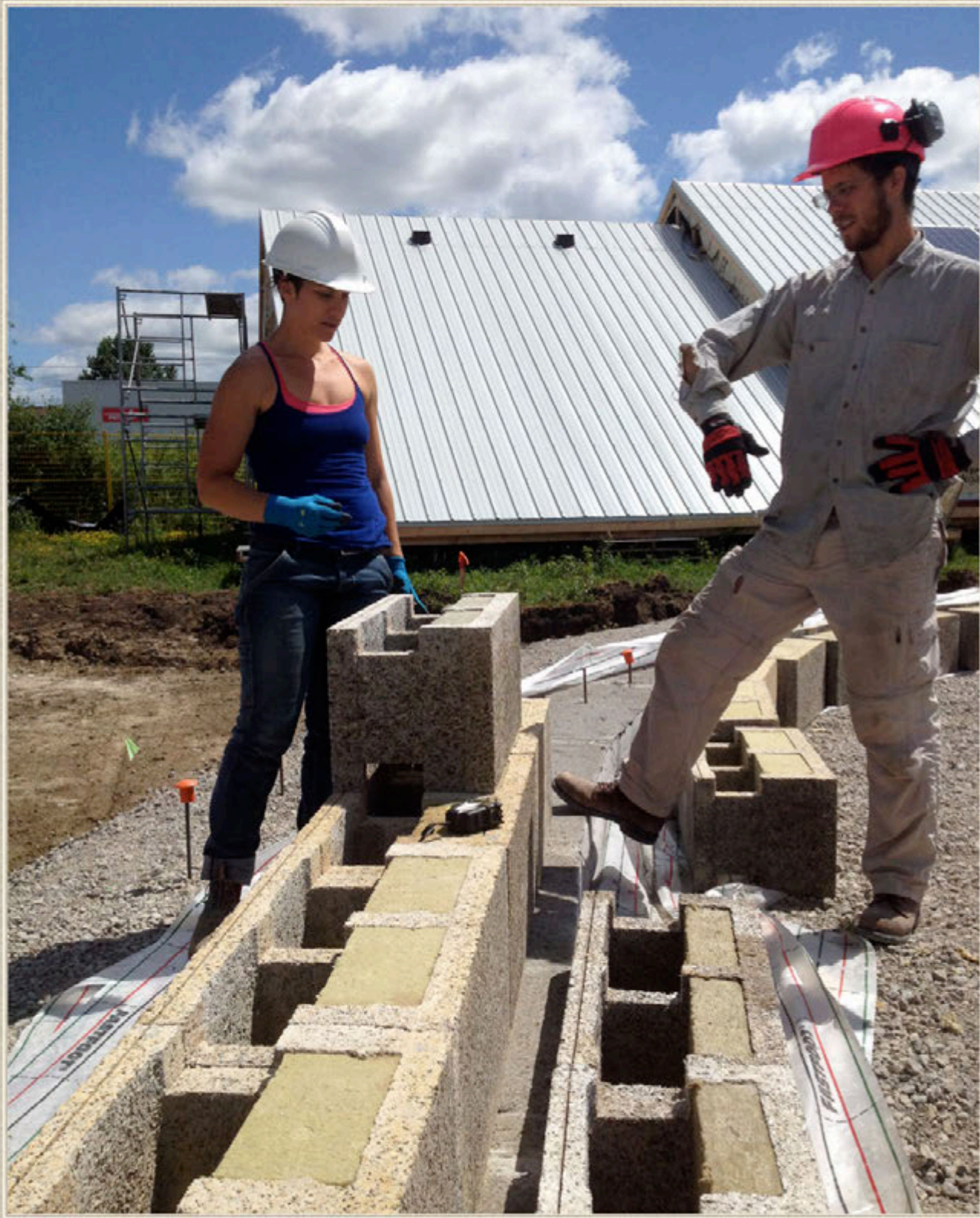
Durisol insulated form blocks are dry stacked . Second course is 2 inches narrower than the first, creating a ledge for the floor joists.
