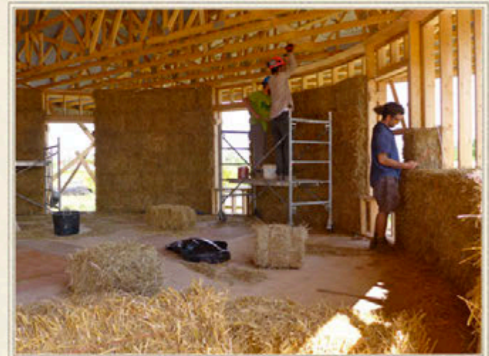
The bale walls go up quite quickly. They easily follow the curved form of the end walls.
