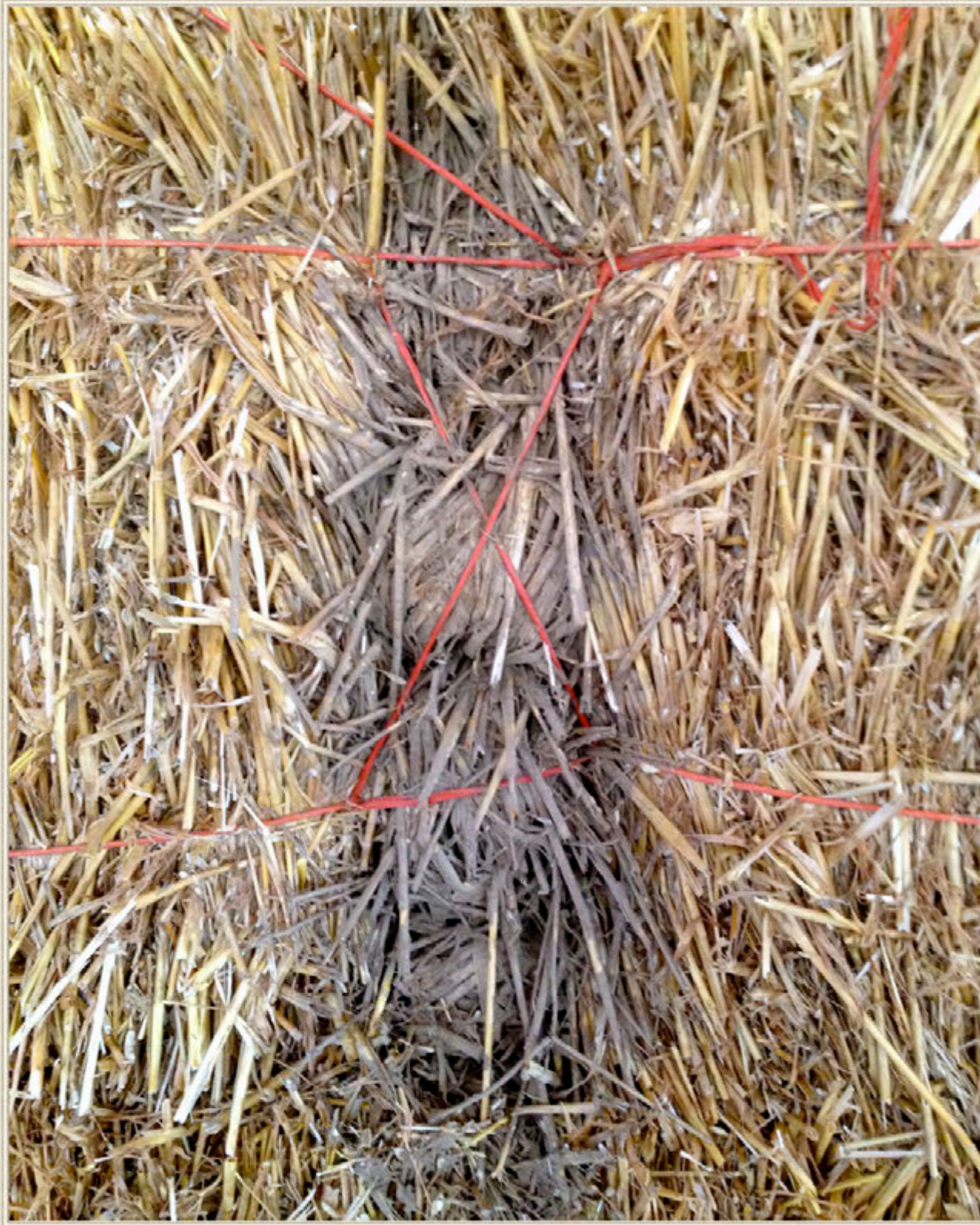
Detailing includes stuffing and lashing joints and taking care of air sealing at all seams using air barriers and mesh.
