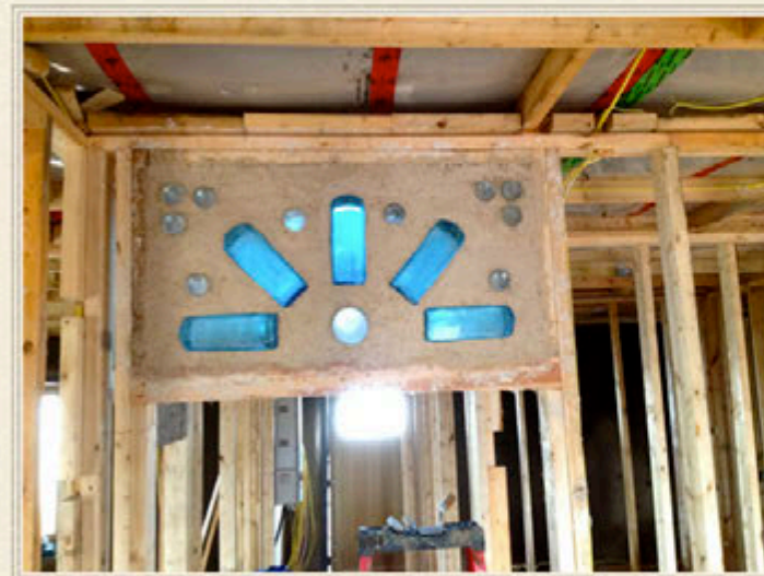
Hempcrete and glass bottles are used to make custom transoms above all the office doorways.
