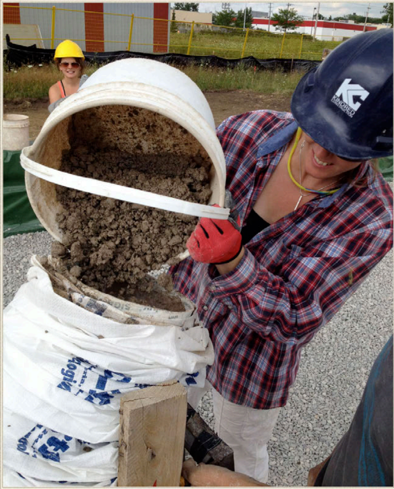
A gravel and homemade hydraulic lime mix is poured into the earthbags and tamped firmly to create a stable foundation wall.
