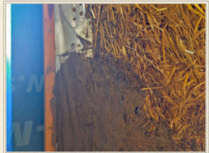
Our first experience using Siga tape to air seal at junctions was a success that we will repeat on future buildings.
