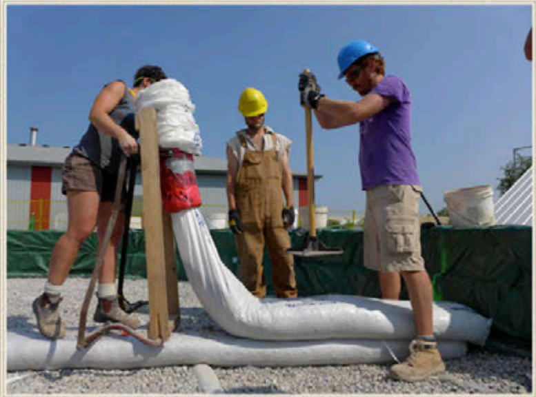
A gravel and homemade hydraulic lime mix is poured into the earthbags and tamped firmly to create a stable foundation wall.
