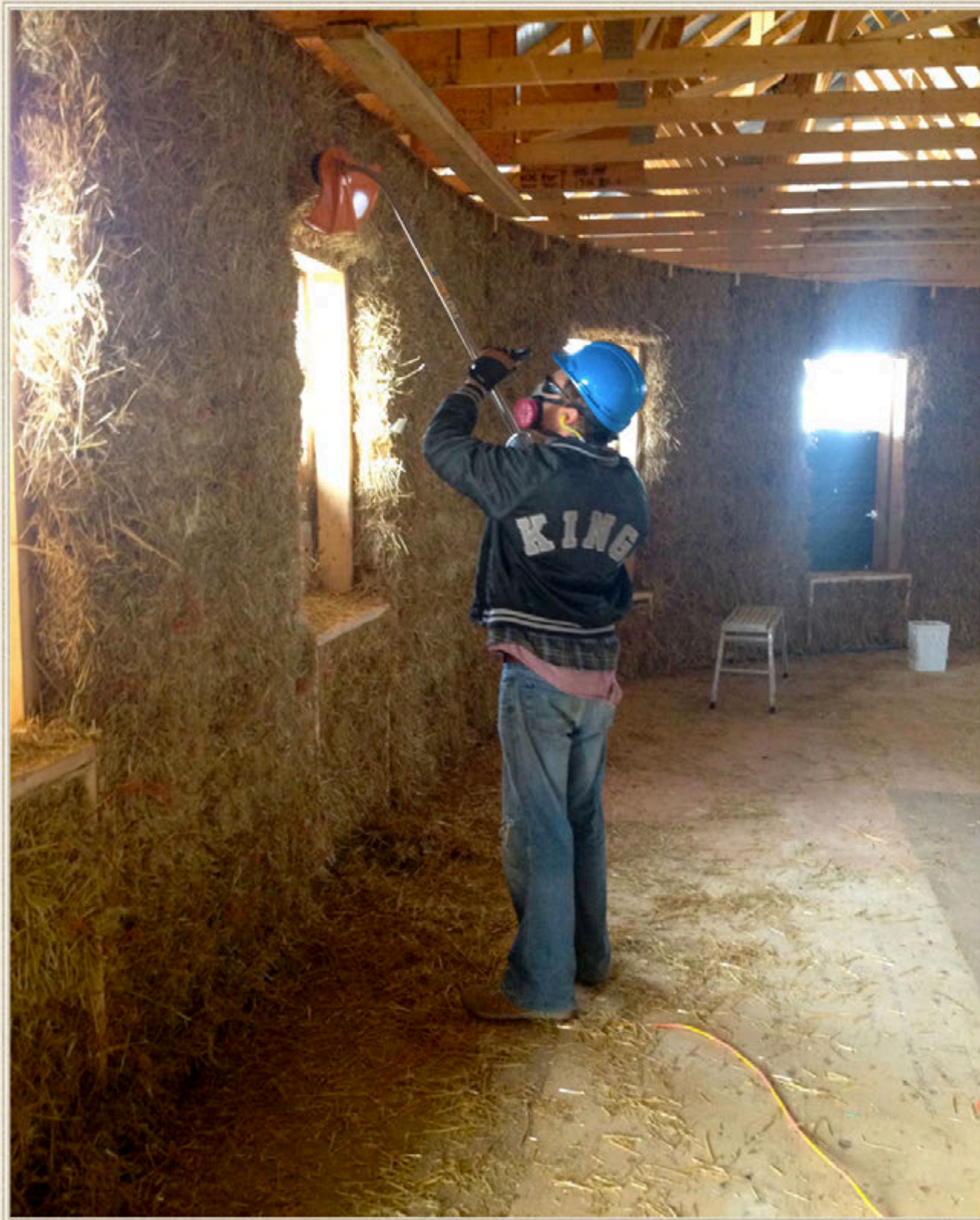
Preparing bales walls for plastering takes much longer than stacking them. Trimming, stuffing gaps with straw/clay and plumbing them all take time.
