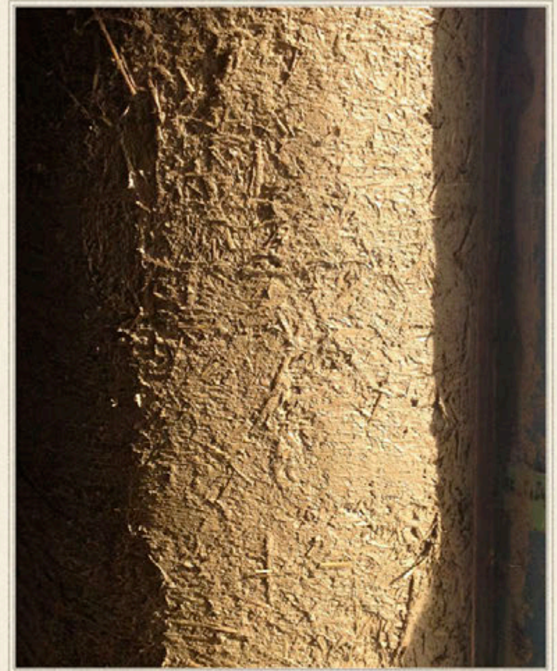
Hand applied earthen plaster is placed in a single thick coat of 1-2 inches .
