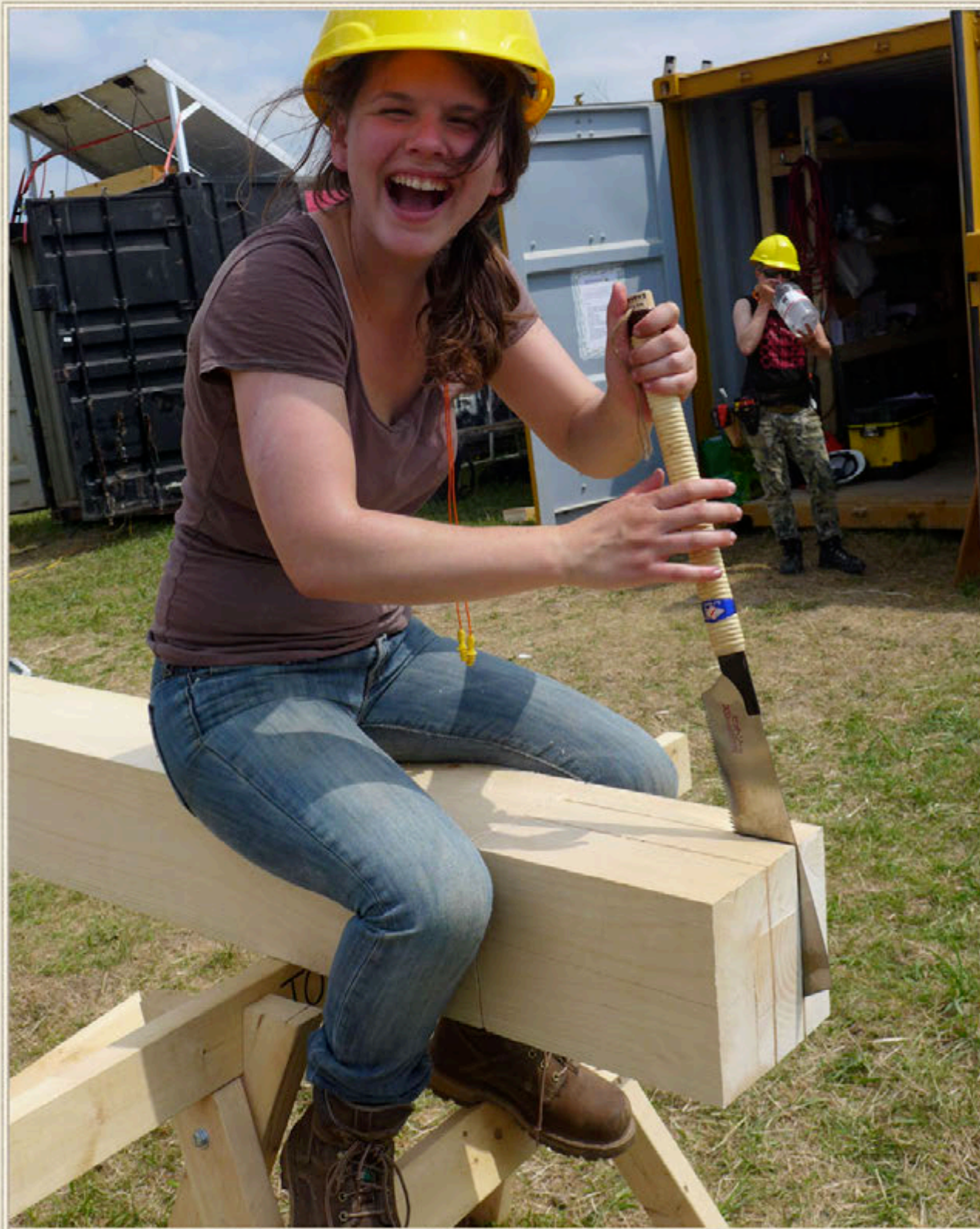
Site work begins with building the four timber frame sections for the corners of the building, using locally harvested and milled white pine timbers.
