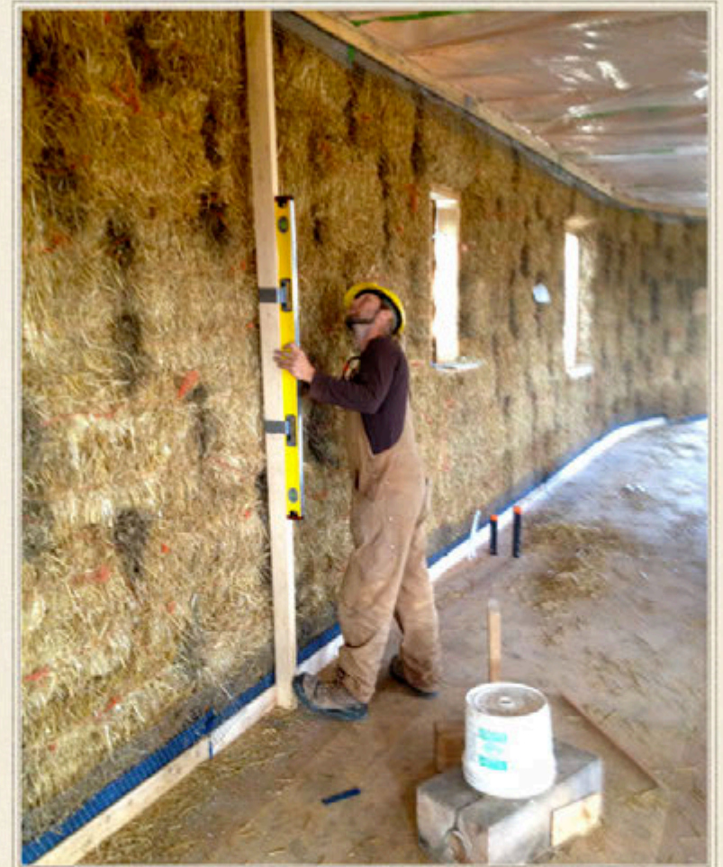
Preparing bales walls for plastering takes much longer than stacking them. Trimming, stuffing gaps with straw/clay and plumbing them all take time.
