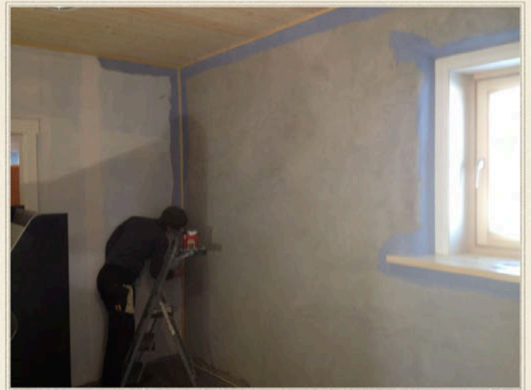
Natural clay paints are used over the clay plaster to provide a final colour.
