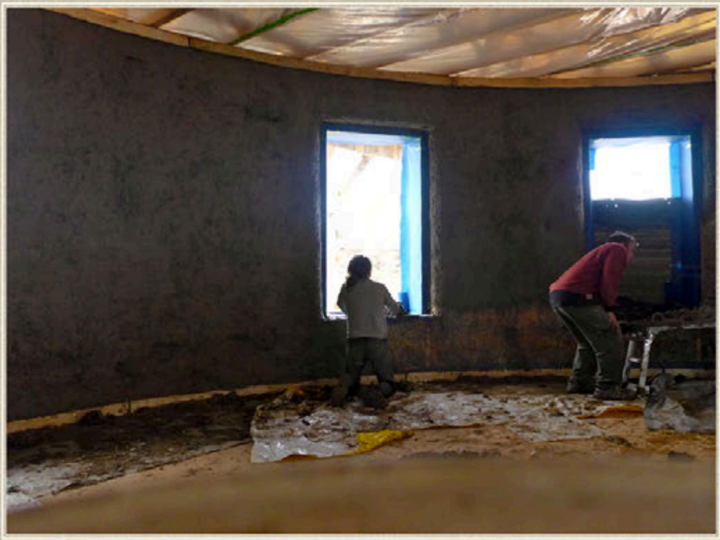
Coordinated team work gets a lot of plastering done in a reasonable amount of time, from push-in layer to floated finish.
