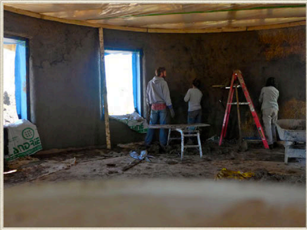
Coordinated team work gets a lot of plastering done in a reasonable amount of time, from push-in layer to floated finish.
