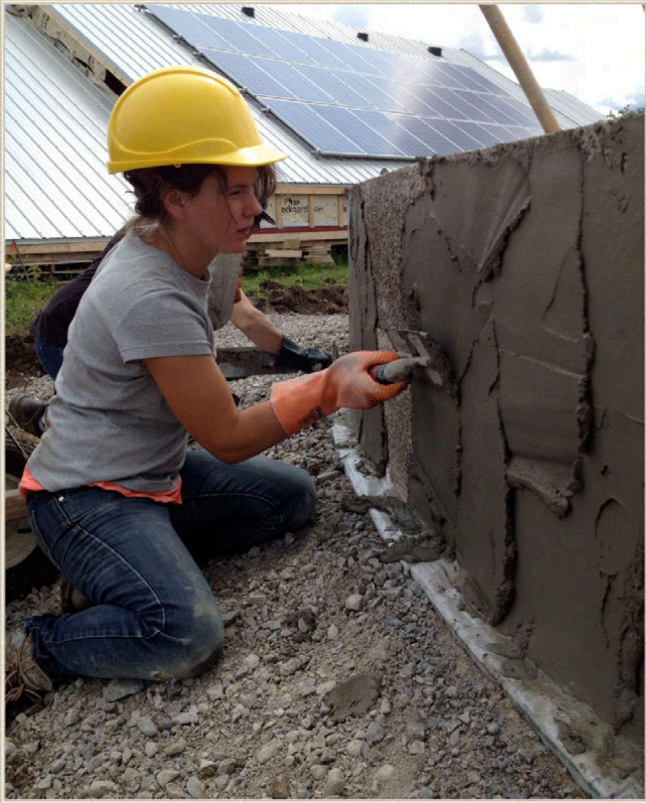
Parging for the exterior of the foundation and a 10 mil poly vapour barrier for the inside provide moisture protection in these two zones.
