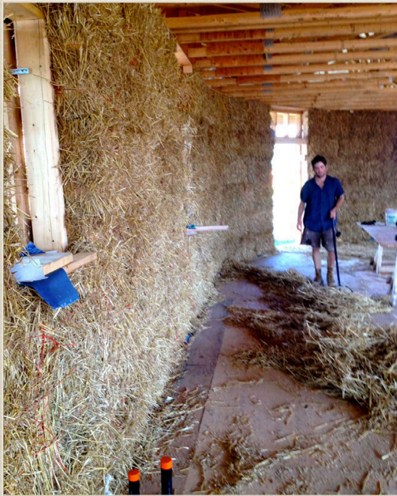
The bale walls go up quite quickly. They easily follow the curved form of the end walls.
