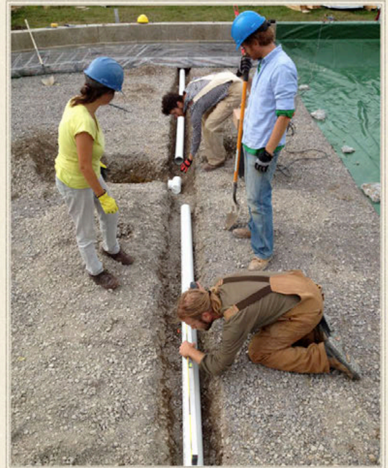
A drainage sump is installed inside the foundation to remove water in extreme weather circumstances.
