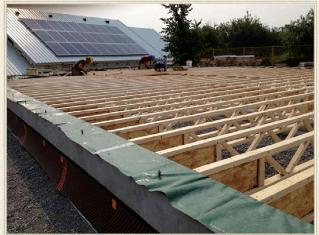
Open web floor joists rest on the Durisol ledge and the earthbag foundation. The vapour barrier is carefully tied in so it joins to the exterior walls.
