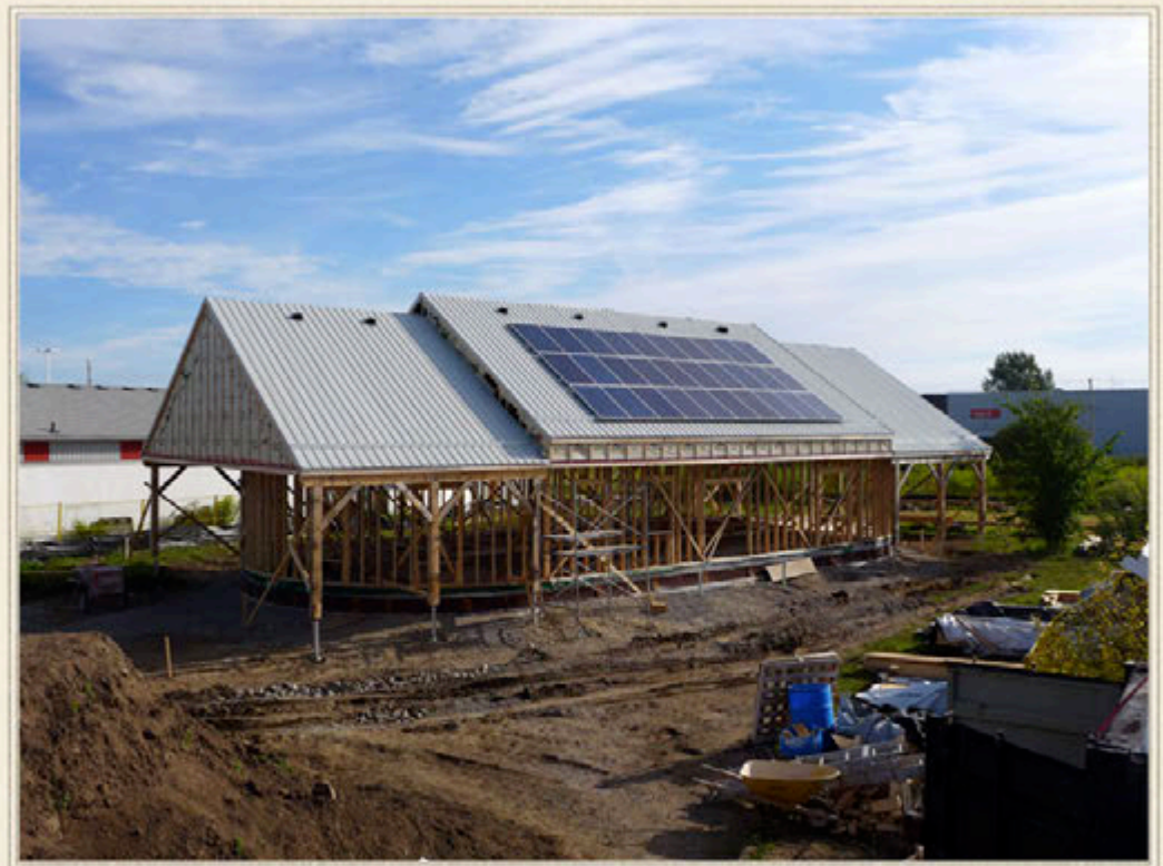
The roof sections are placed and the building is now covered.
