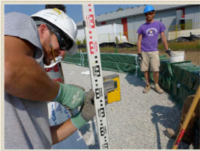
Earthbags are levelled during tamping. Barbed wire goes between courses, and the ends of bags are folded under.
