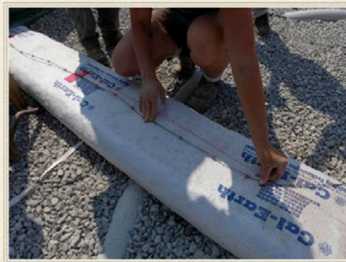
Earthbags are levelled during tamping. Barbed wire goes between courses, and the ends of bags are folded under.
