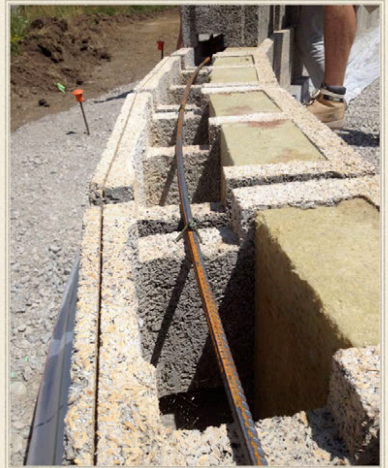
Durisol insulated form blocks are dry stacked . Second course is 2 inches narrower than the first, creating a ledge for the floor joists.
