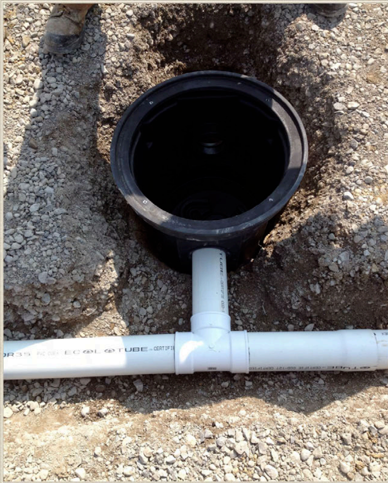
A drainage sump is installed inside the foundation to remove water in extreme weather circumstances.
