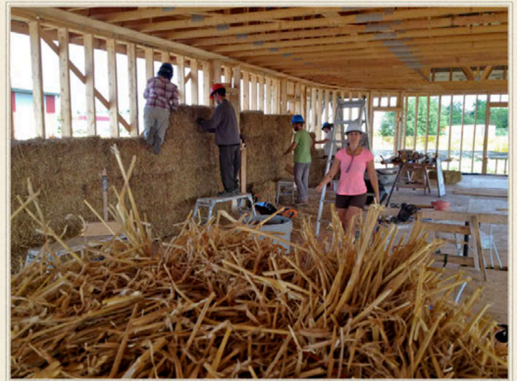
Raising straw bale walls is always a highlight of a build!
