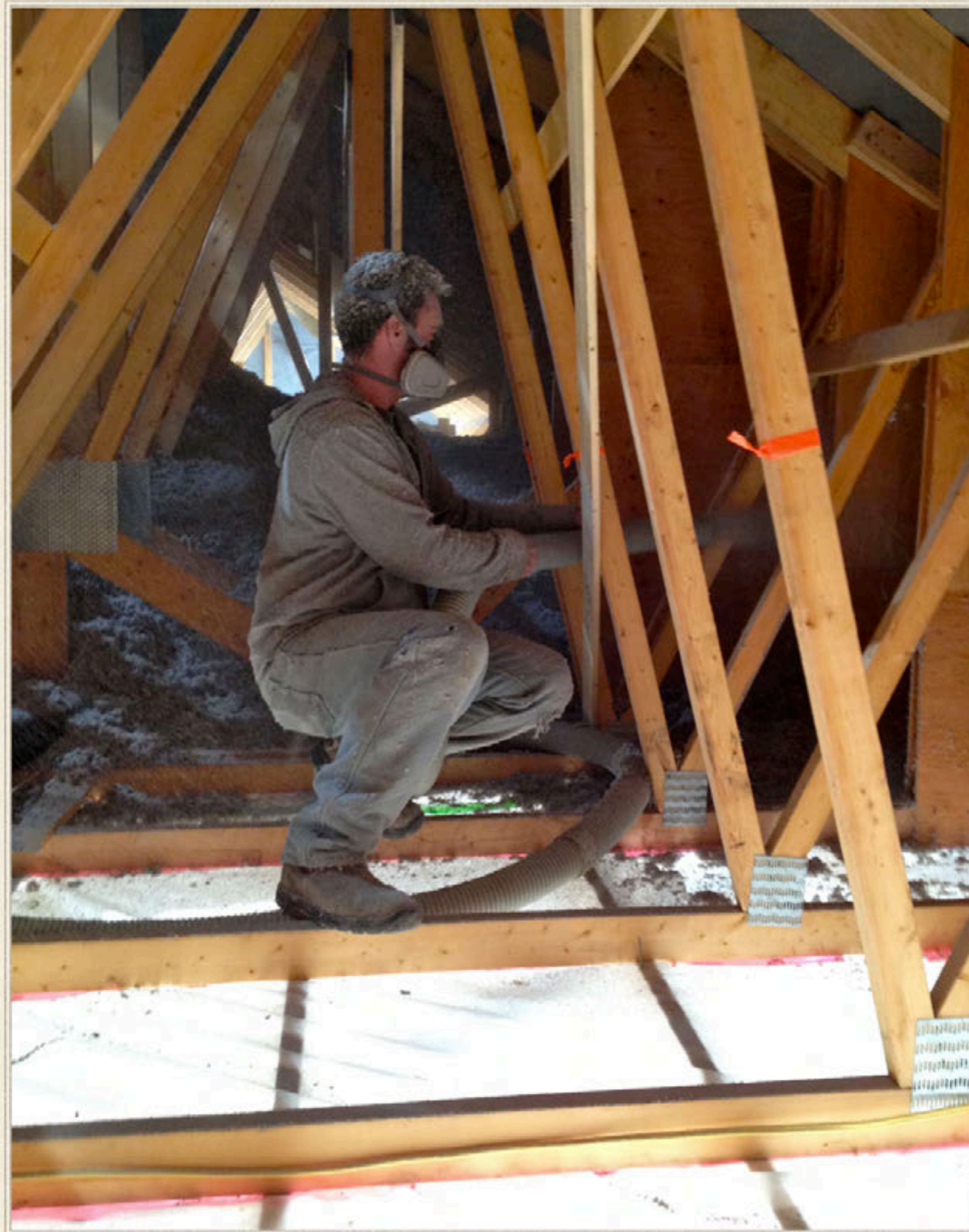
Cellulose is blown into the attic to R-1000.
