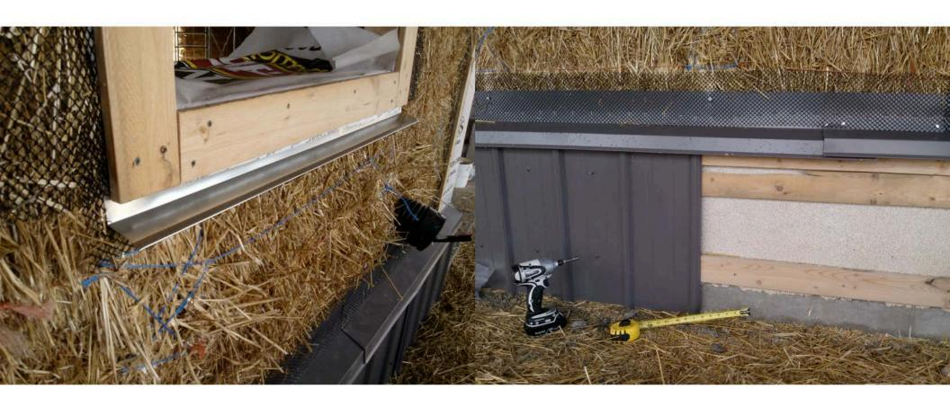
The walls are prepared for plastering, which includes flashing and meshing around windows and over the metal base flashing that covers the Poraver foundation.
