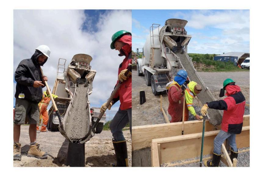
High slag content concrete is poured into the pier tubes and into the foundation forms, creating a 4 inch thick footing to support the Poraver foundation.
