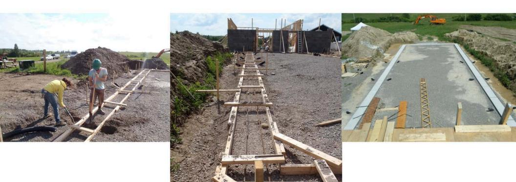
With the framing nearly completed for the first story, the formwork for the quonset hut root cellar footing is completed.
