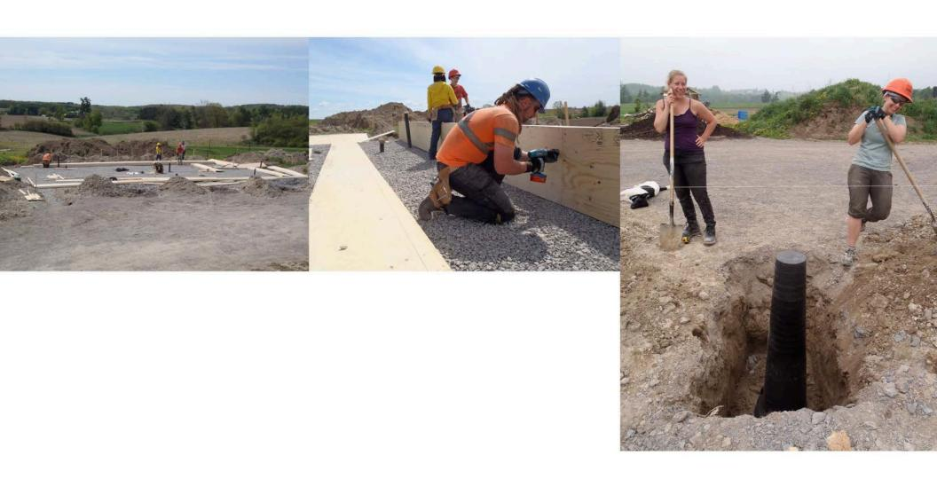
Formwork is constructed on the gravel pad for the Poraver foundation. Pier tubes are dug to support the timber frame on the north side of the building.
