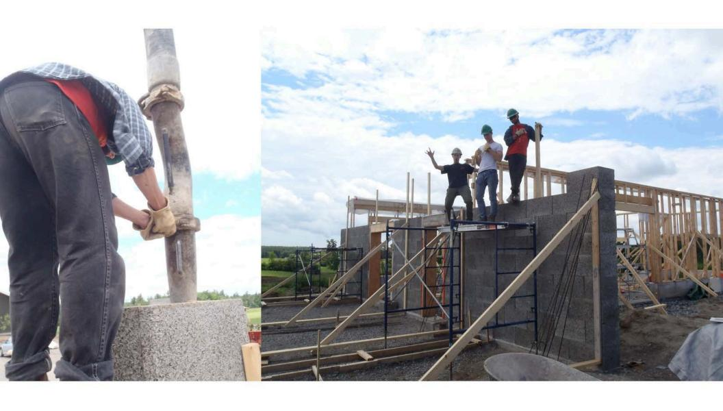
A concrete pumper truck is used to core fill the Durisol blocks. In very short order, the first floor height of the Durisol wall is completed.
