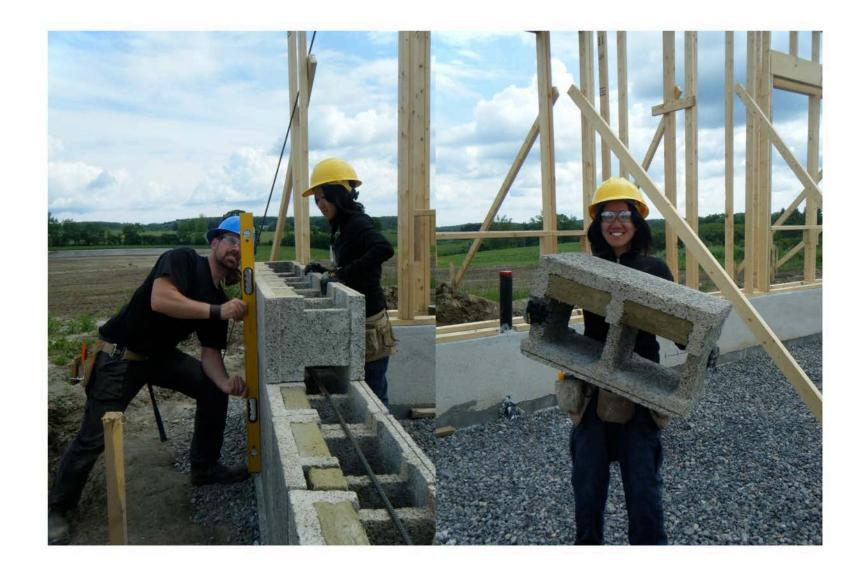
Durisol blocks begin to form the dividing wall between the processing building and the root cellar. The blocks are dry stacked and the cores poured with high slag concrete.
