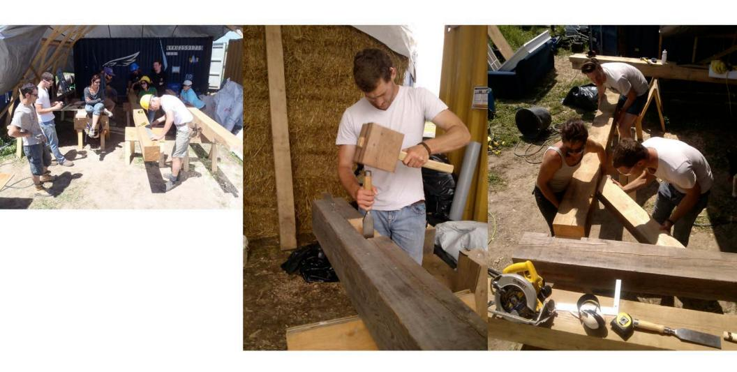
The timber frame for the north porch is cut and fit in the shelter next to the building. Instructor Mark Davidson provided the basics, and the class completed the frame.
