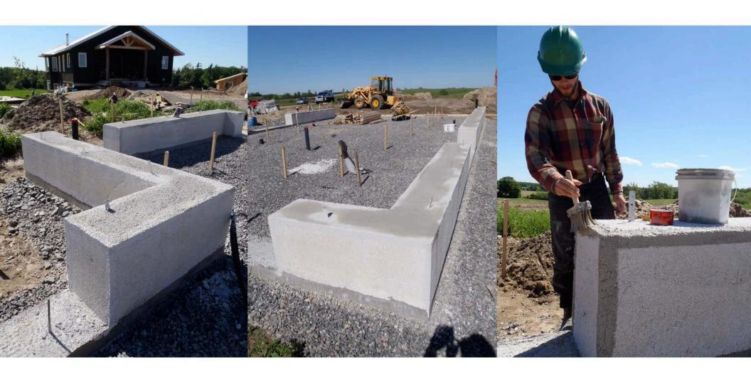
The formwork is stripped from the foundation wall after 24 hours. The hydraulic reaction of the lime/metakaolin mixture ensures that it is set. Kevin paints slip on the edges to help bind them and protect from damage.
