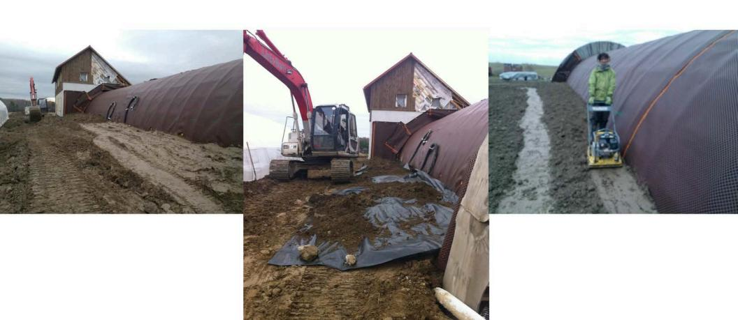
Soil is backfilled against the quonset hut. Ventilation tubes are placed to provide air supply to the storage areas. Each lift of backfill is compacted. Keeping loads balanced is important!
