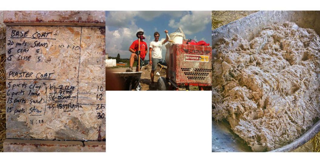
A new type of plaster is made from the same ingredients as the foundation binder. It uses hydrated lime and metakaolin with a very high percentage of chopped straw.
