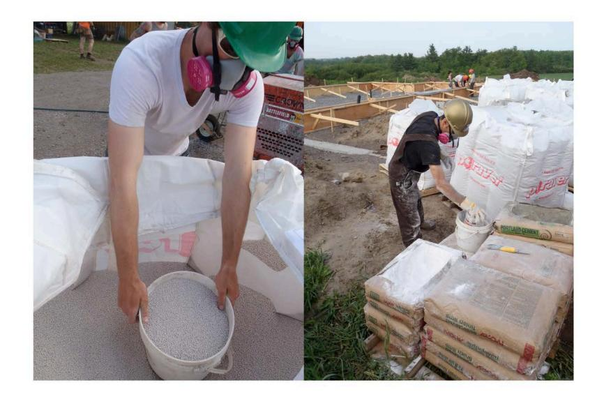
Poraver is an expanded glass bead project made from recycled glass. Very lightweight yet strong, the beads are cast with a binder made from hydrated lime and metakaolin, which is a byproduct of the glass bead manufacturing process.
