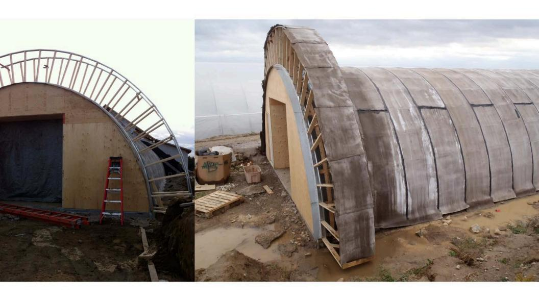
A rounded "parapet" is created to hold back the soil that will be placed on the quonset hut. It too is covered with concrete cloth.
