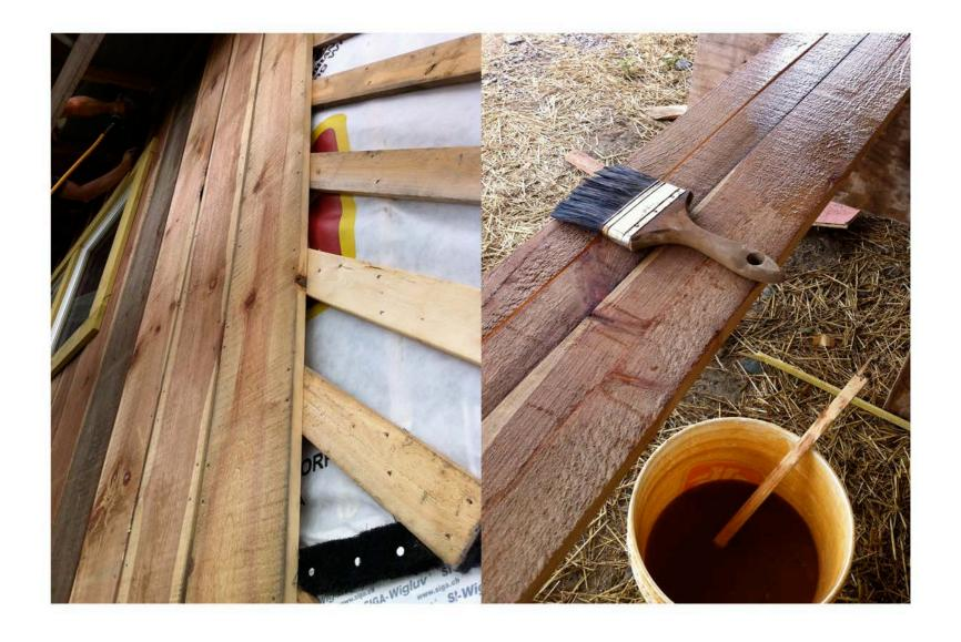
"Lifetime" is a mineral protectant used on the wood siding on the upper floor of the building. The board and batten siding is fastened to angled strapping to provide bracing and ventilation behind the siding.
