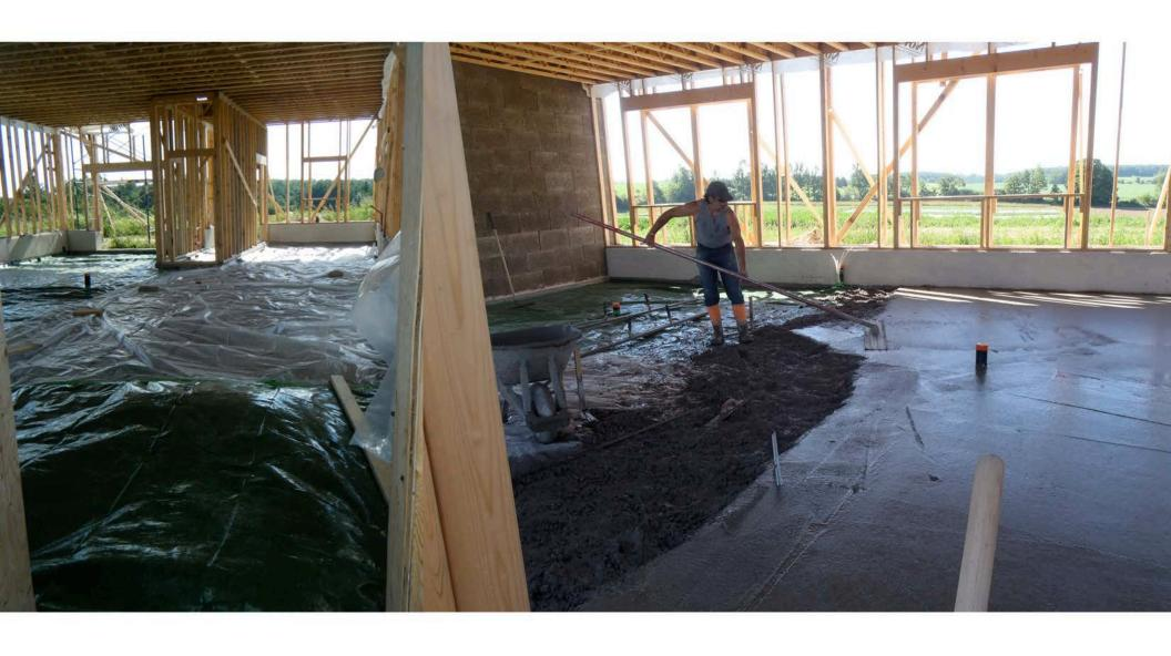
A heavy 10 mil poly vapour barrier is placed on the floor area and caulked to the Poraver foundation. A high slag concrete slab is poured on the main floor.
