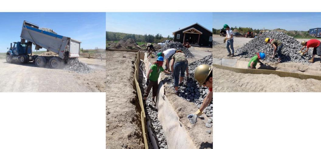
A larger crushed stone (4 inch) was used in the rubble trench. This proved very difficult to move by hand/shovel, so a loader was used to fill the trench.
