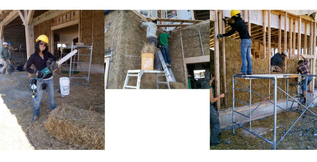
Melissa handles custom bale sizing with an electric chainsaw while the rest of the crew fill up each wall with bales.
