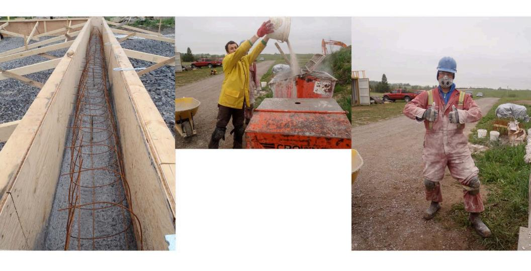
Wire mesh is bent into a "cage" to provide tensile strength inside the Poraver stem wall. Bart oversees the mixing process, while Gord demonstrates appropriate safety gear for the job.
