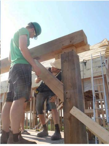
The north side timber frame is assembled on the pier foundation. Rough cut hemlock rafters are cut to rest on the hemlock frame.
