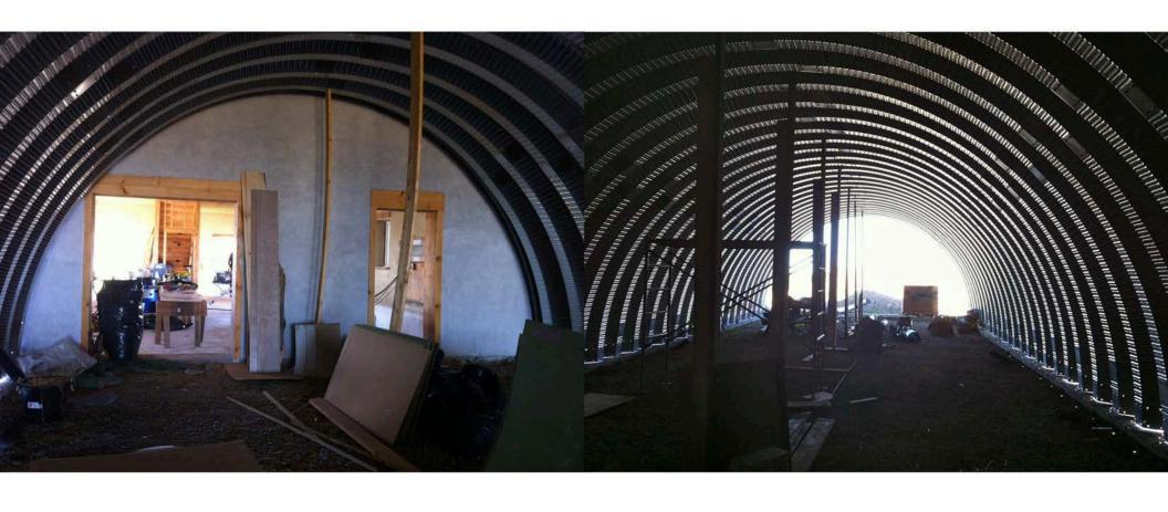
The quonset hut sections are bolted together to form the 80 foot length of the root cellar.
