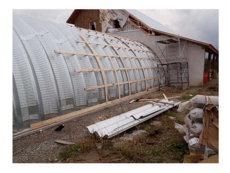
The main building is nearly complete. The quonset hut receives a double layer of wooden strapping to support the concrete cloth covering that strengthens and waterproofs the cellar.
