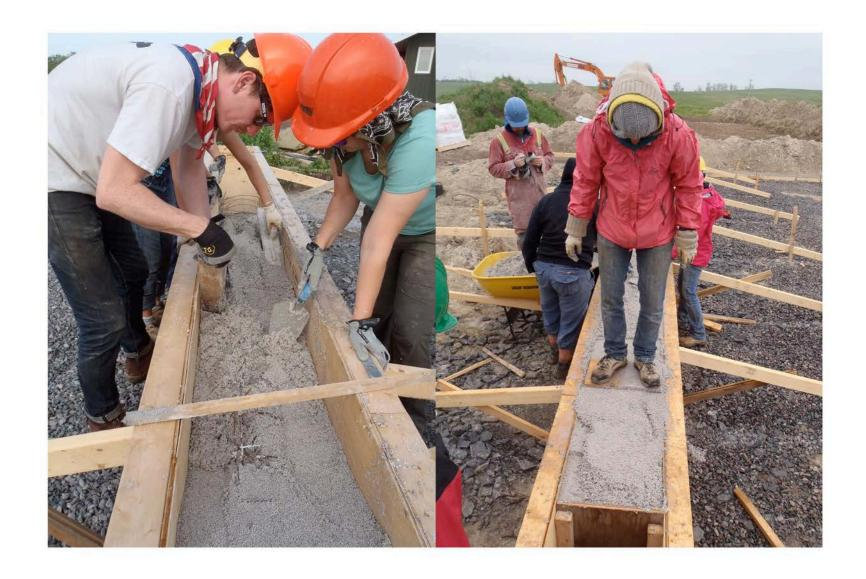
The Poraver mix is quite dry and requires manual tamping to ensure an even density without air pockets. Lara provides her body weight to flatten the top surface.
