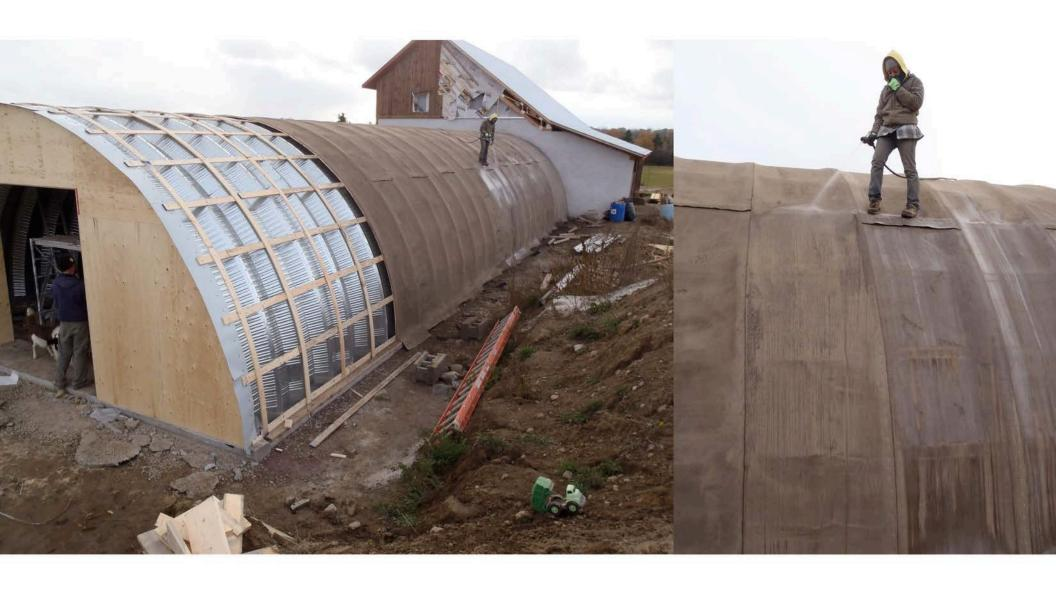
The concrete cloth is laid over the strapping and then sprayed down with water to activate the hydraulic setting of the concrete embedded in the canvas.
