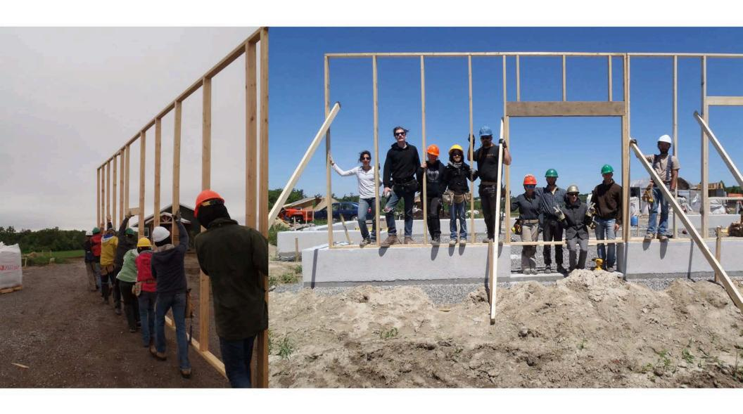
Wall framing begins in earnest, the sections having been built during the foundation forming process. The 2x4 double frames go up quickly.
