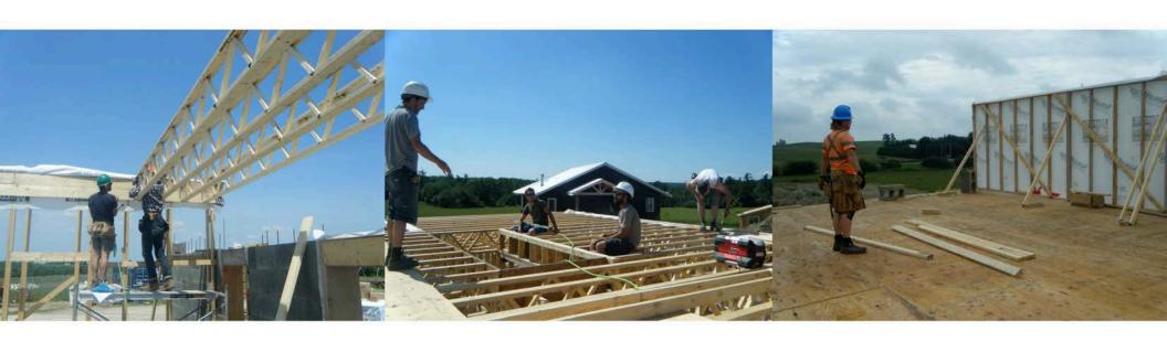
Second floor framing begins with open web joists and a plywood deck. Second floor walls are framed and raised on this platform.
