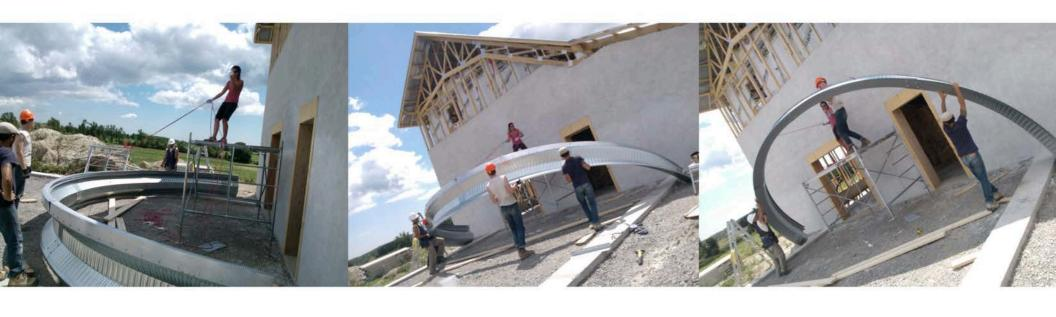
The quonset hut that will form the root cellar begins to be installed. Each prefab metal arch is assembled on the ground and then lifted into place.
