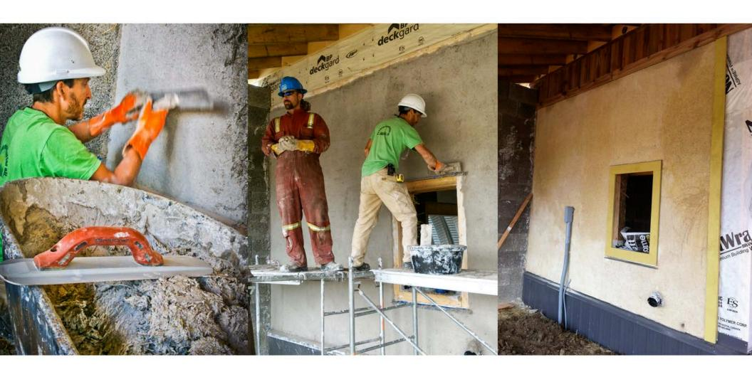
The plastering process involves preparing the surface with a no-straw mix, into which the high-straw mixed is pressed by hand. Floats are used to smooth surface. One thick coat is all that is required.
