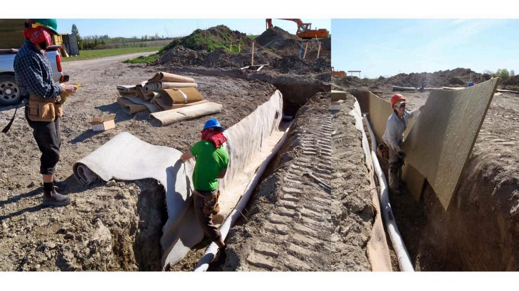
Used carpet lines the dig for the trench, providing a barrier between the soil and the rubble and some insulation value. Roxul drainboard (right) can serve the same purposes.
