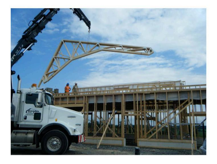
The roof trusses arrive and are placed on the second floor deck. The crew frames them up and braces them. The open south face and the protected northern exposure are now formed.
