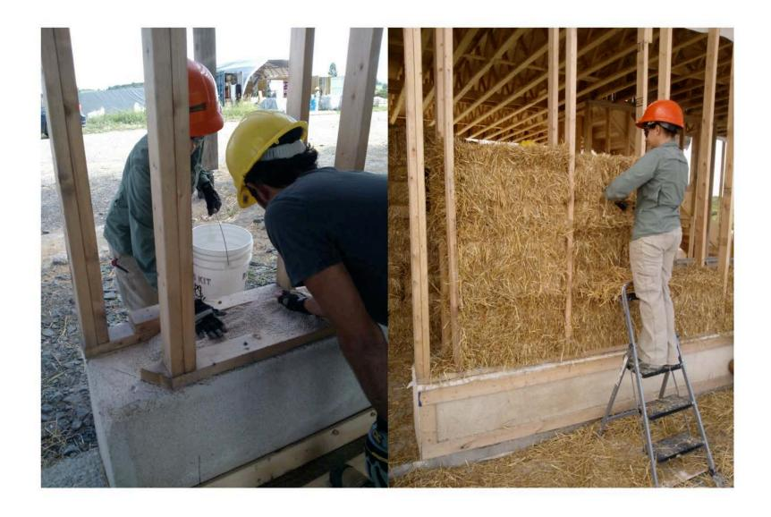
The straw bales arrive and the space between the two stud frames is insulated with loose Poraver in preparation. The bales are inserted in stud cavities that are one bale in length.
