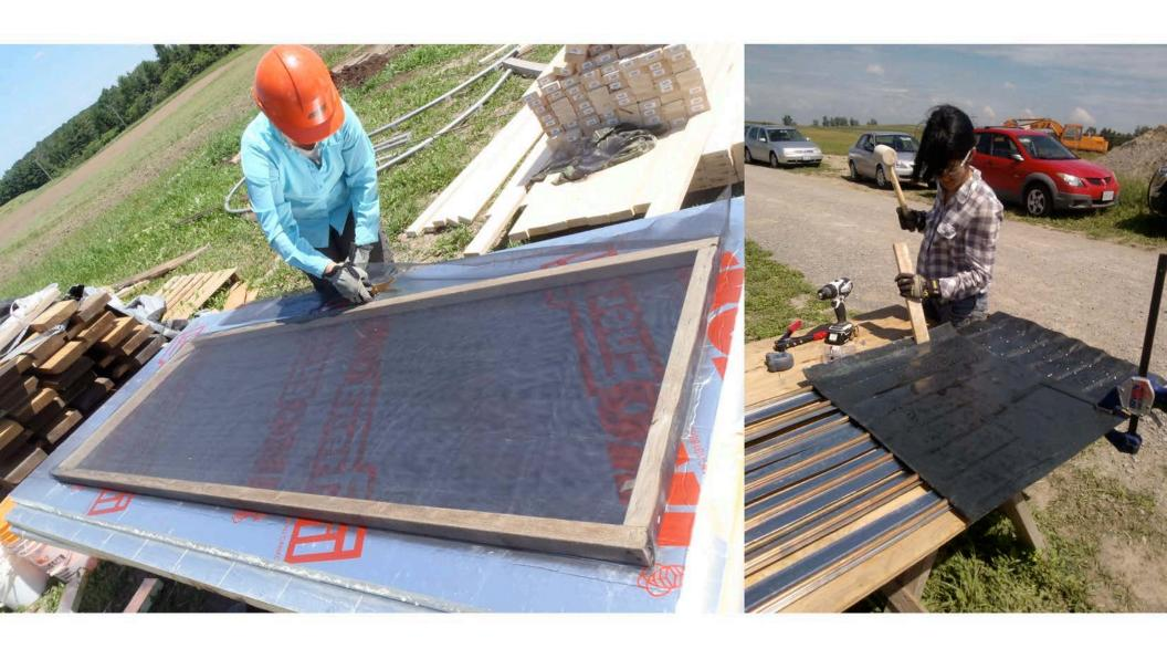
Two layers of screen force air to move through the mesh and get warmed on the air collectors. Copper pipe has used copper sheet form fitted to increase water collector area.
