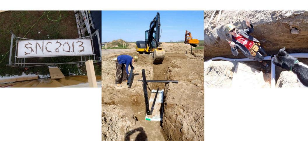
Despite some late season snow, the digging of the rubble trench foundation gets underway. Earth tube ventilation pipes and drainage tiles are laid in the bottom of the trench
