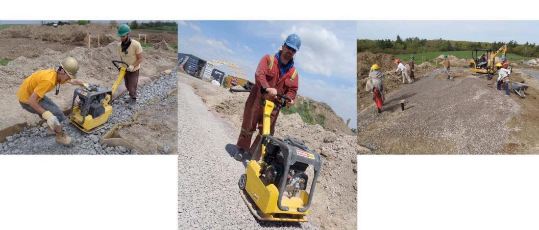
The 4 inch rubble is compacted into the trench until it reaches existing grade. A layer of 3/4 inch stone is then compacted over the entire foundation area of the building.
