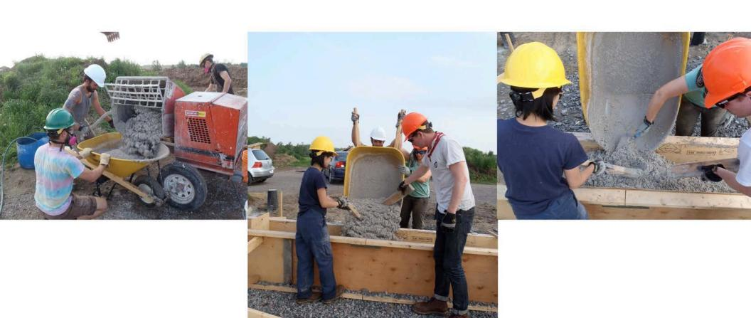
The Poraver mix is emptied from the mortar mixer into wheelbarrows and is brought to the forms, where it is dumped and spread inside the forms.
