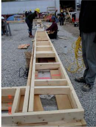
Top plate assembled on the foundation.
