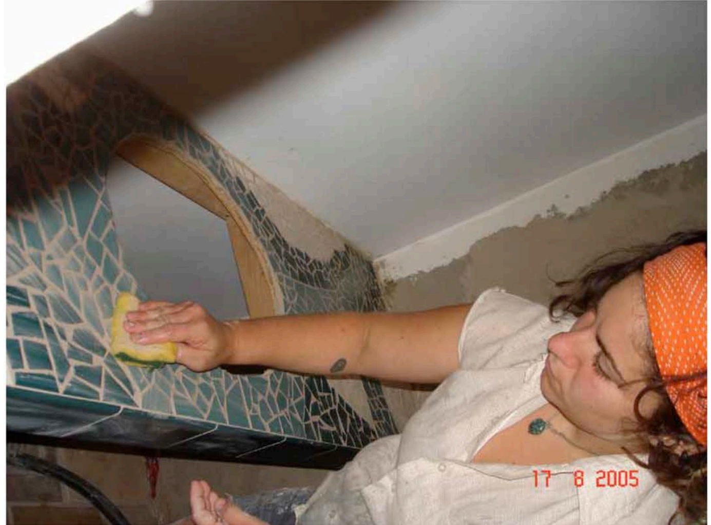
Tiling sink The sink area is given a custom tiling job.
