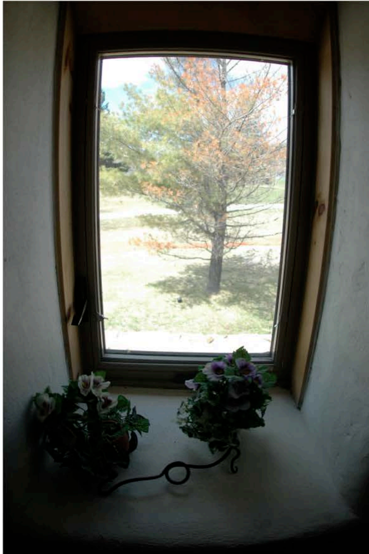
Finished window sill
