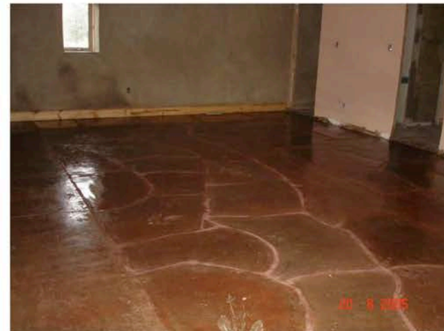
Soil cement floor finish
